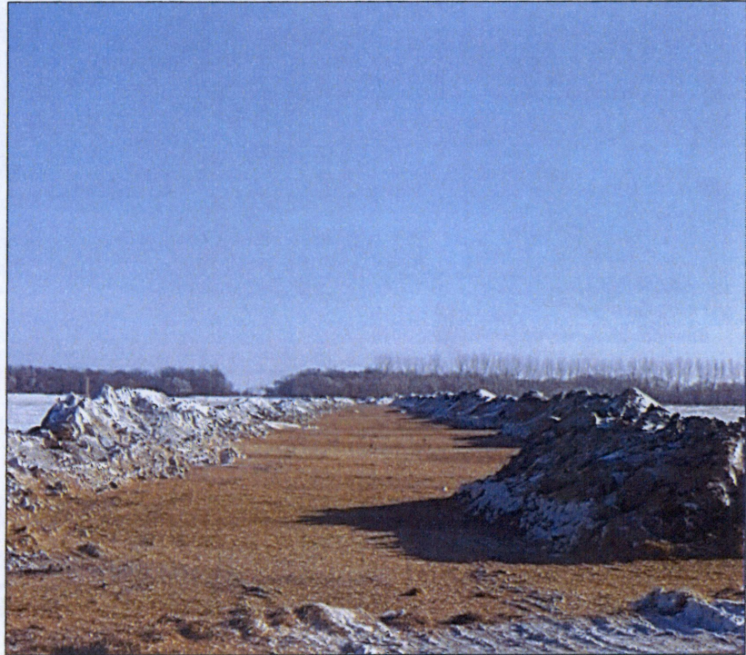
Right-of-Way Prepared for Final Stabilization
