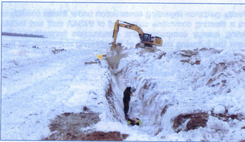
Snow Removal From Trench
