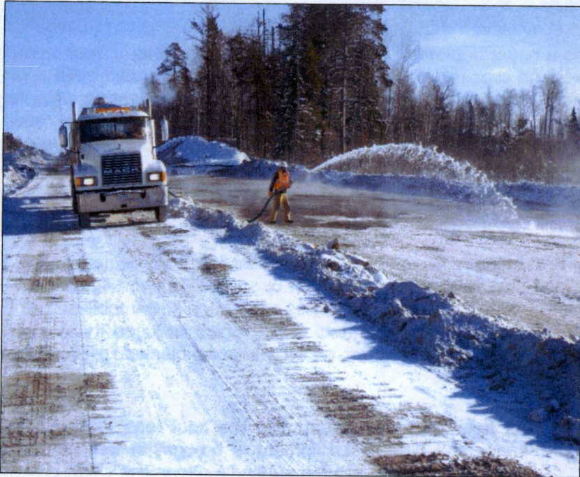
Building the Ice Road
