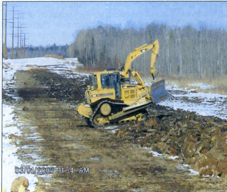
Reducing Frozen Crown Over Backfilled Trench
