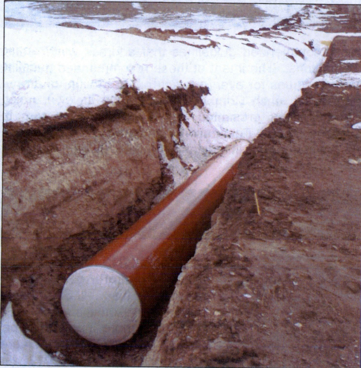
Pipeline Construction in Frozen Conditions
