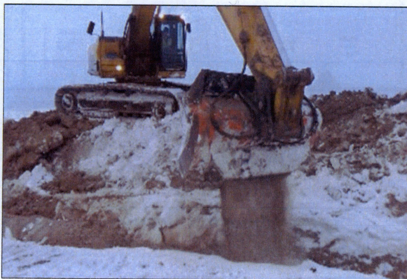
Shaker Equipment Backfilling Trench
