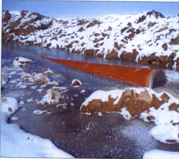
Trench With Frozen Infiltrated Groundwater
