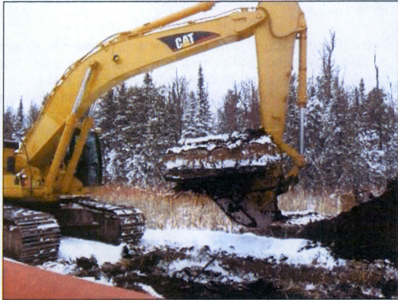
Segregating Frozen Topsoil Layer in Wetland
