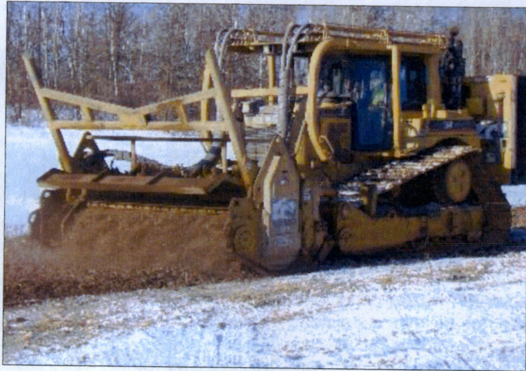
Iron Wolf Breaking up Frozen Topsoil
