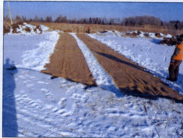
Stabilization of the Right-of-Way
