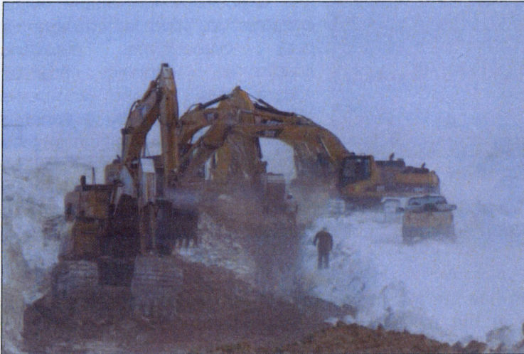
Pipeline Construction in Frozen Conditions
