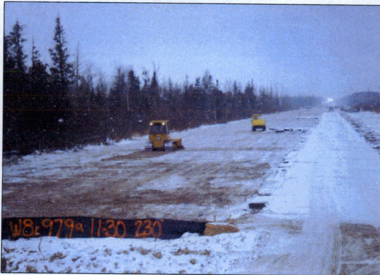
Preparing the Right-of-Way
