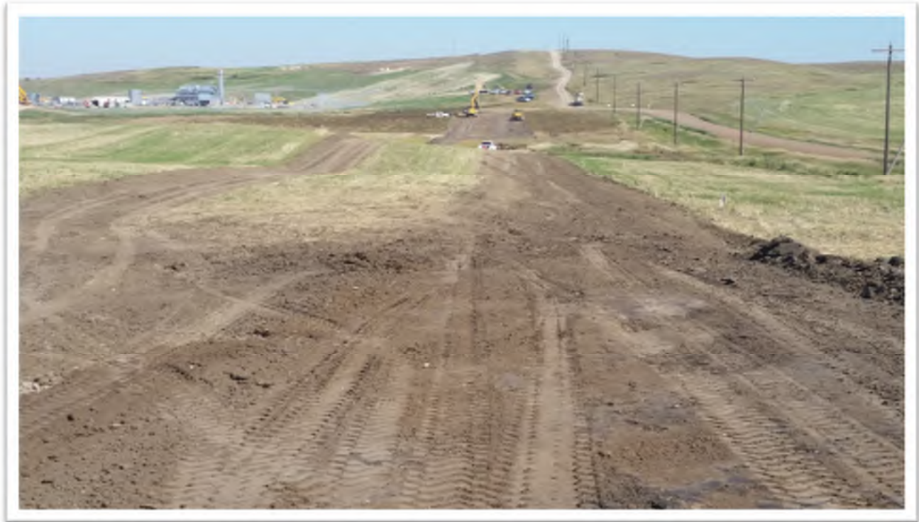
Figure 3. View from pipeline right of way looking north towards WET1.
