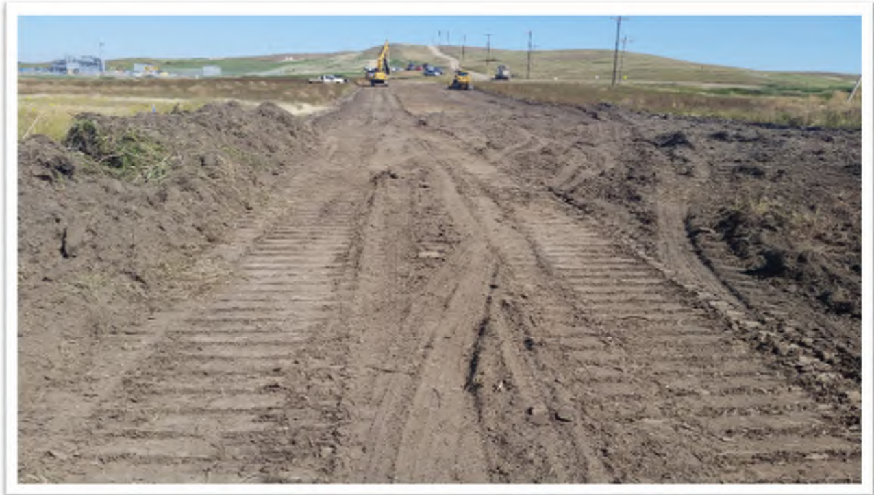
Figure 1. View from northern edge of wetland WET1, looking north. Topsoil removed to County Road 37.
