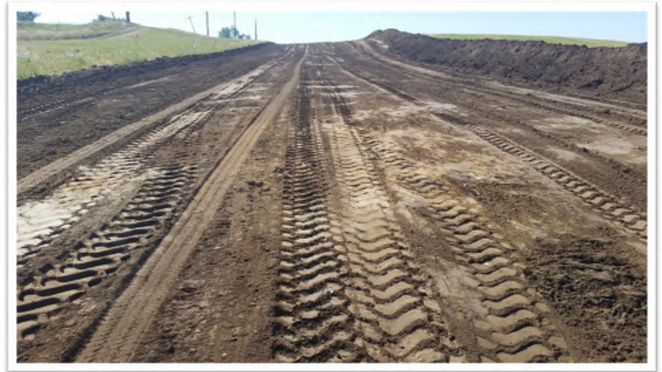
Figure 4. View from pipeline right of way looking south. Topsoil stockpiled along western edge of right of way.
