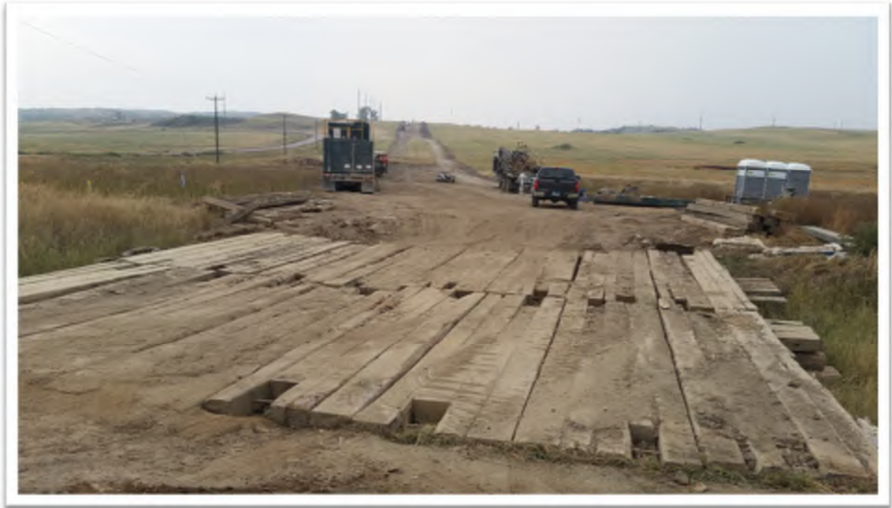
Figure 1. View of right of way progress from County Road 37, looking south.
