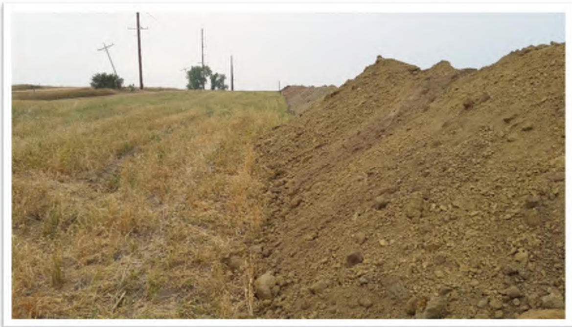
Figure 2. View looking south at subgrade stockpiled within right of way limits.
