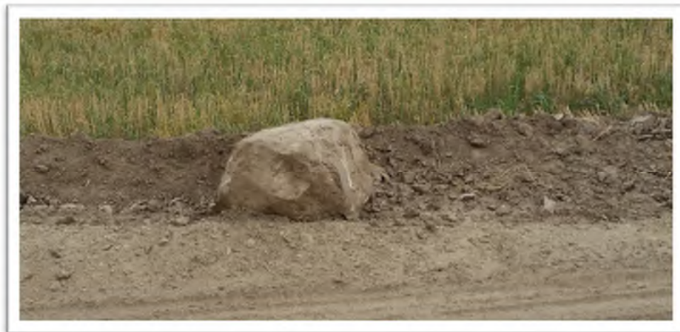
Figure 6. Boulder encountered during topsoil removal operations.
