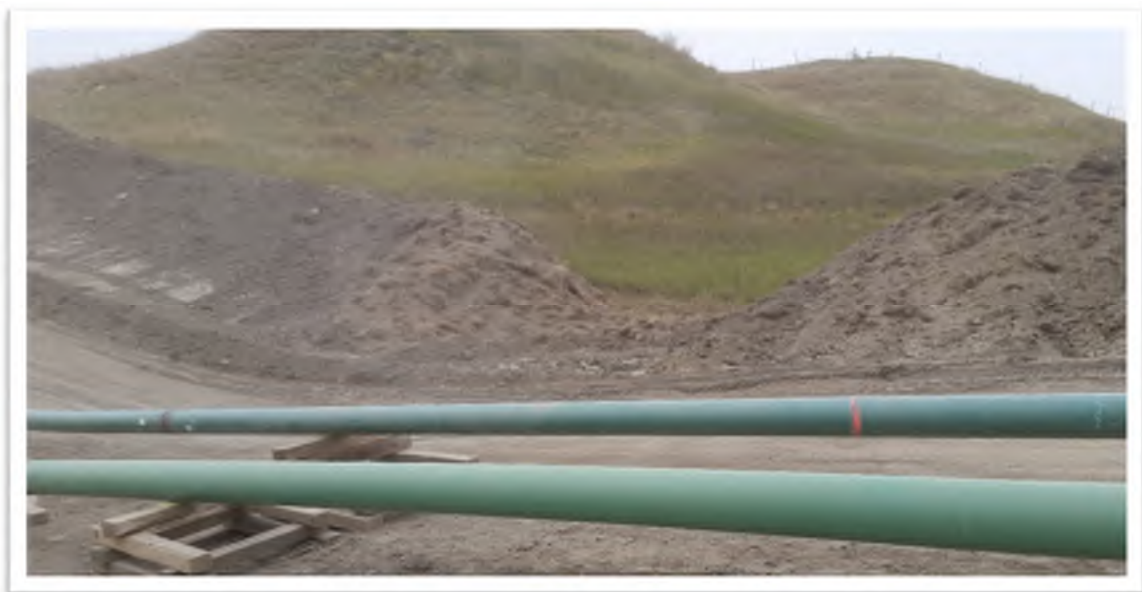
Figure 8. Drainage swale cut out of topsoil stock pile.
