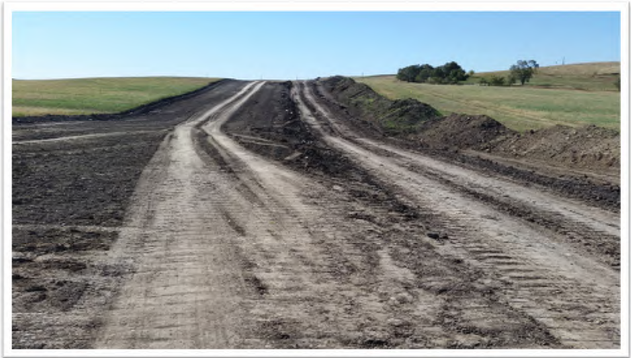
Figure 3. View of subgrade blended back into original contours looking west.
