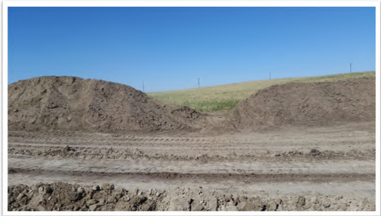
Figure 5. Drainage swale cut out of topsoil stock pile.
