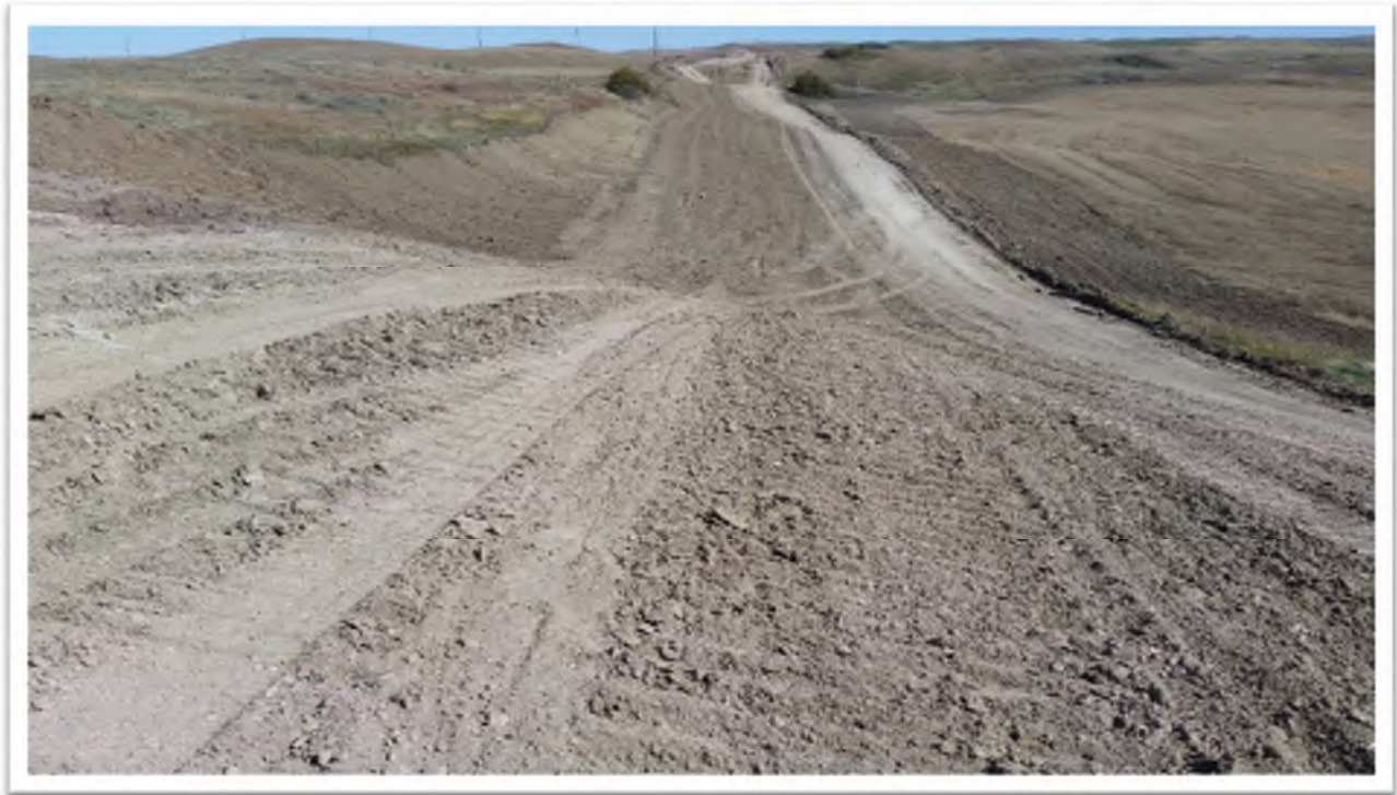
Figure 7. View of subgrade blended back into original contours looking east.
