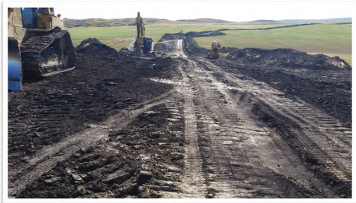
Figure 2. View of subgrade blended back into original contours looking south.
