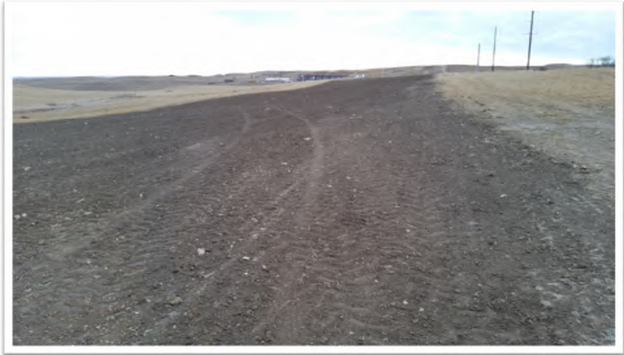
Figure 1. View of agricultural land topsoil blended back into original contours looking north.
