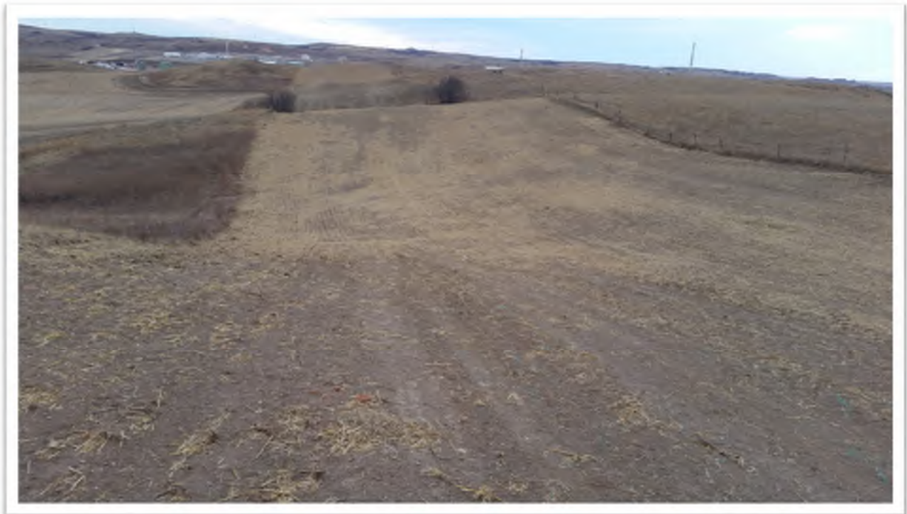
Figure 6. View of grass land topsoil blended back into original contours looking west.
