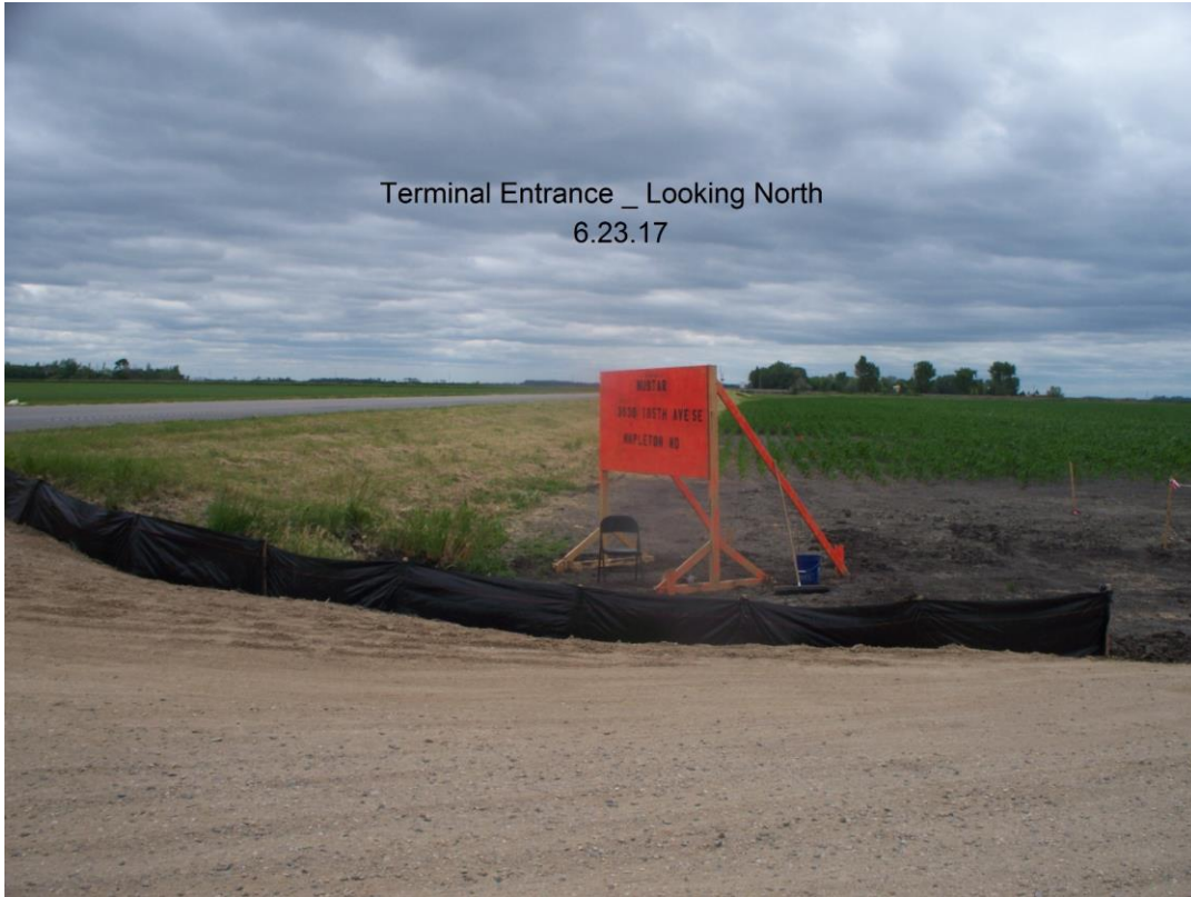
Terminal entrance looking north
