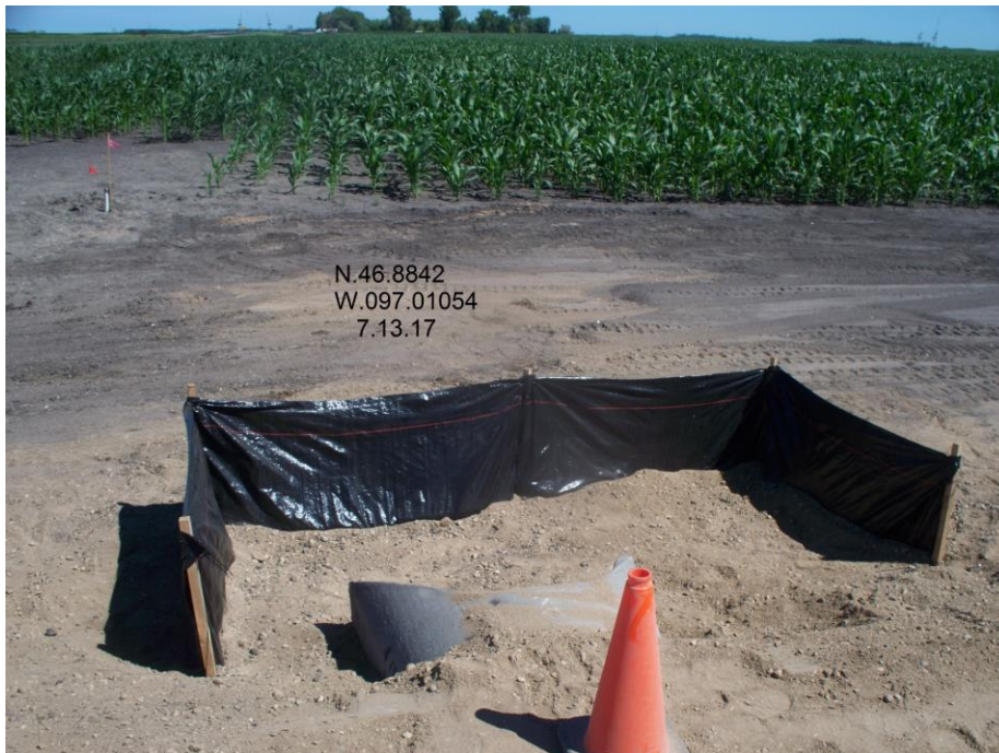
West culvert installation with silt fence
