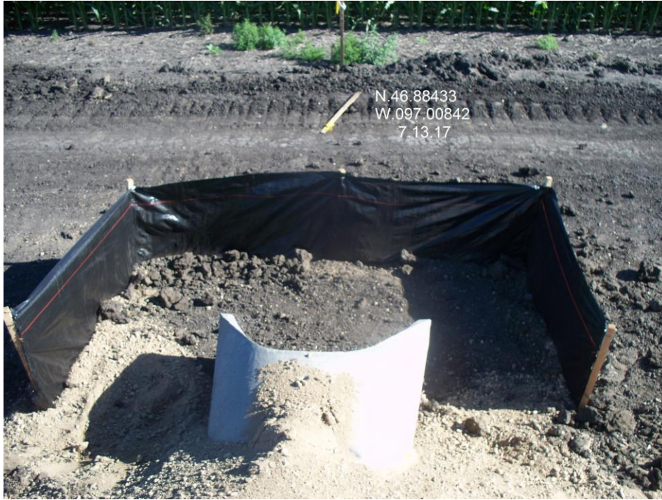
East culvert installation with silt fence
