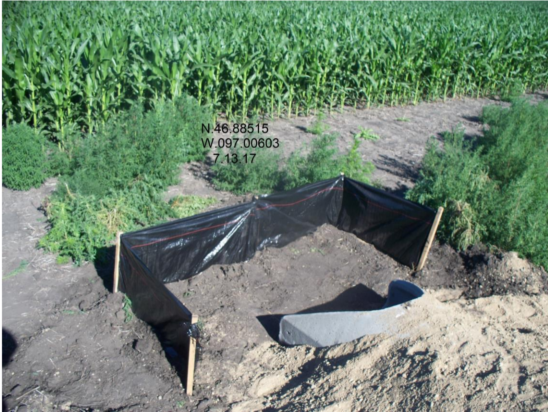
North culvert with silt fence
