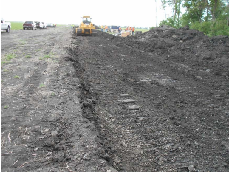
Photo 24: Topsoil separation.
