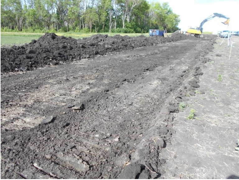
Photo 26: Topsoil separation.
