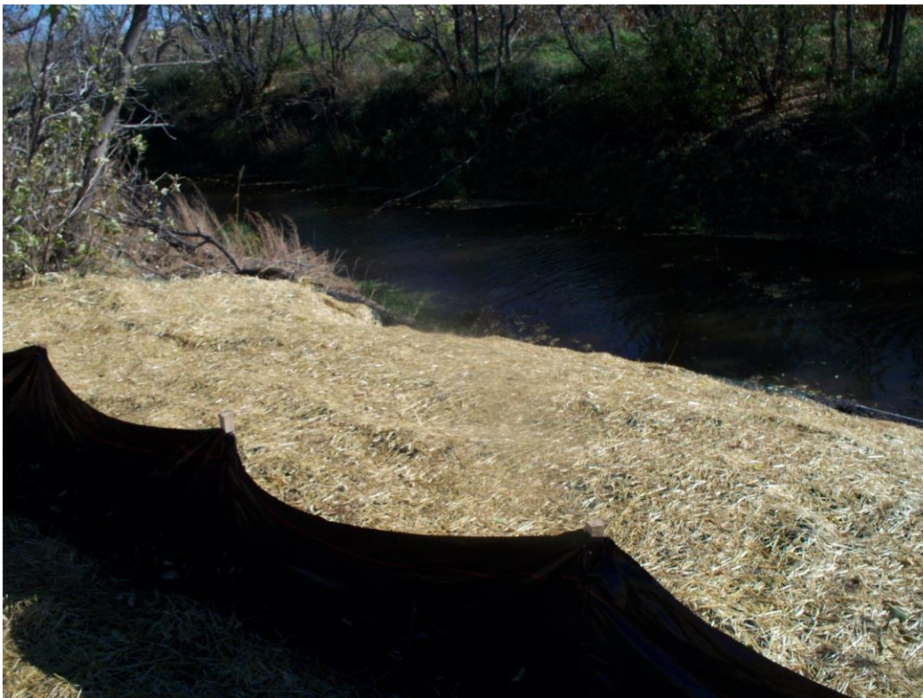
Silt fence, erosion control blanket, and tributary to Sheyenne River
