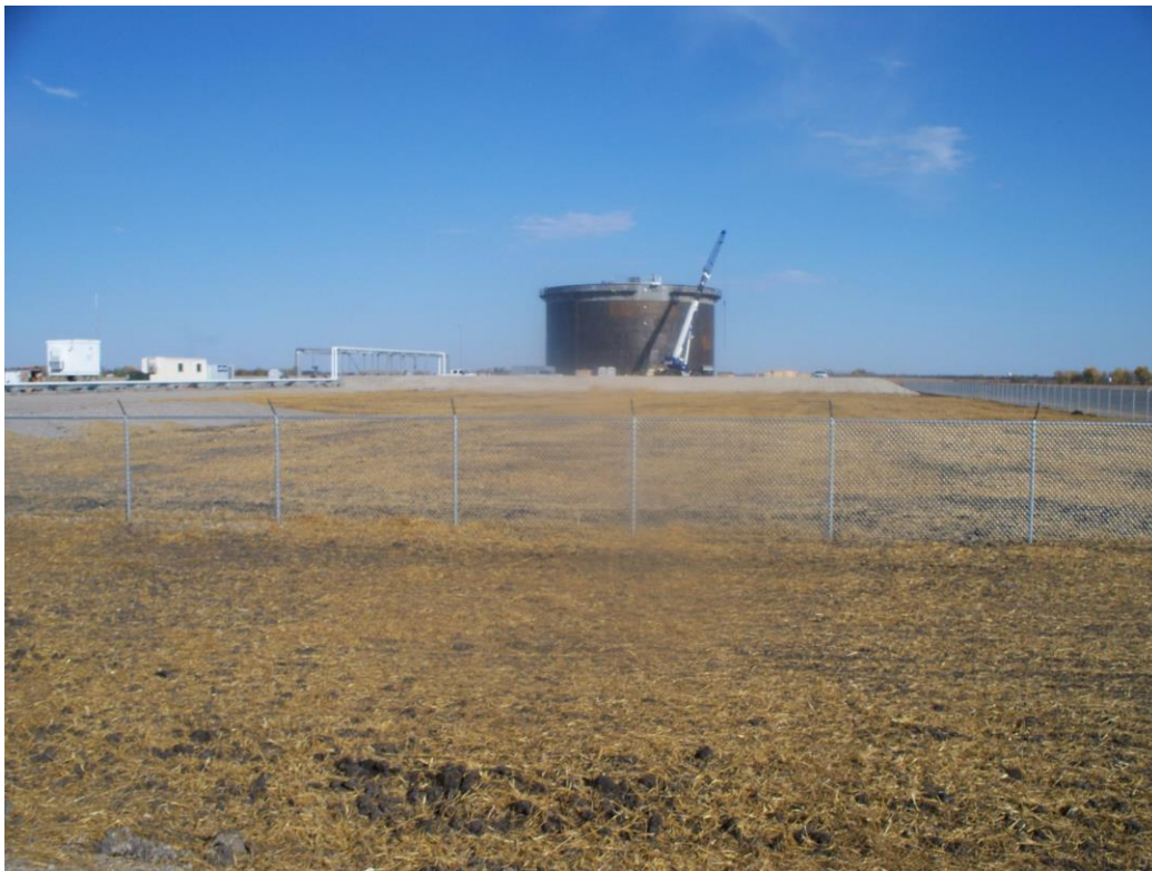
Tank construction nearing completion; seeding of terminal site, looking east.
