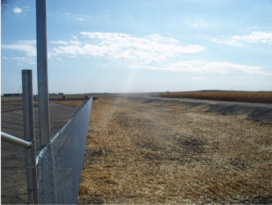
Seeding/mulching at terminal site; 165 th Avenue to the right, looking south.
