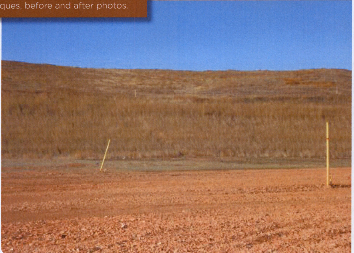
Final restoration with erosion control structures removed
