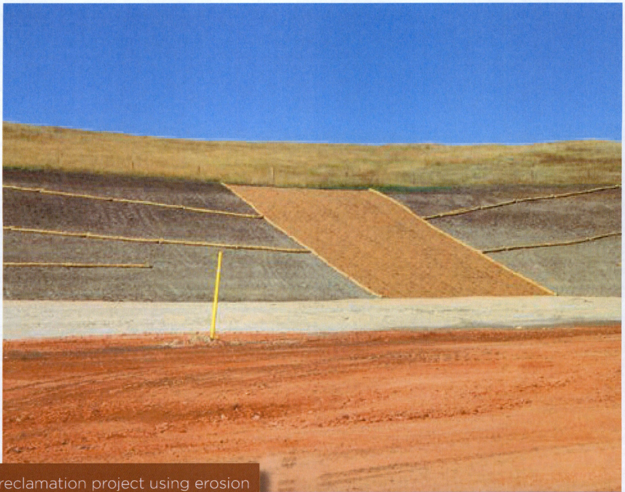
Erosion control during the reclamation process
