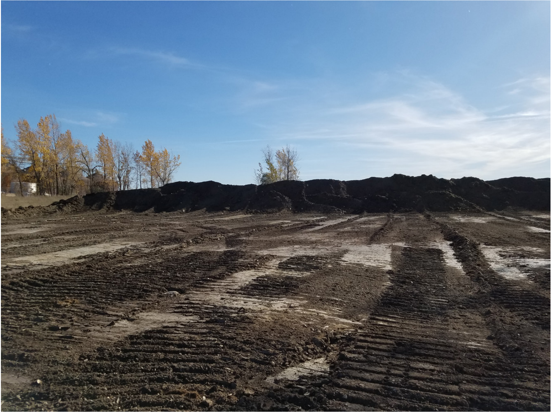
Photo 10 - Topsoil stockpile on south edge of site looking south
