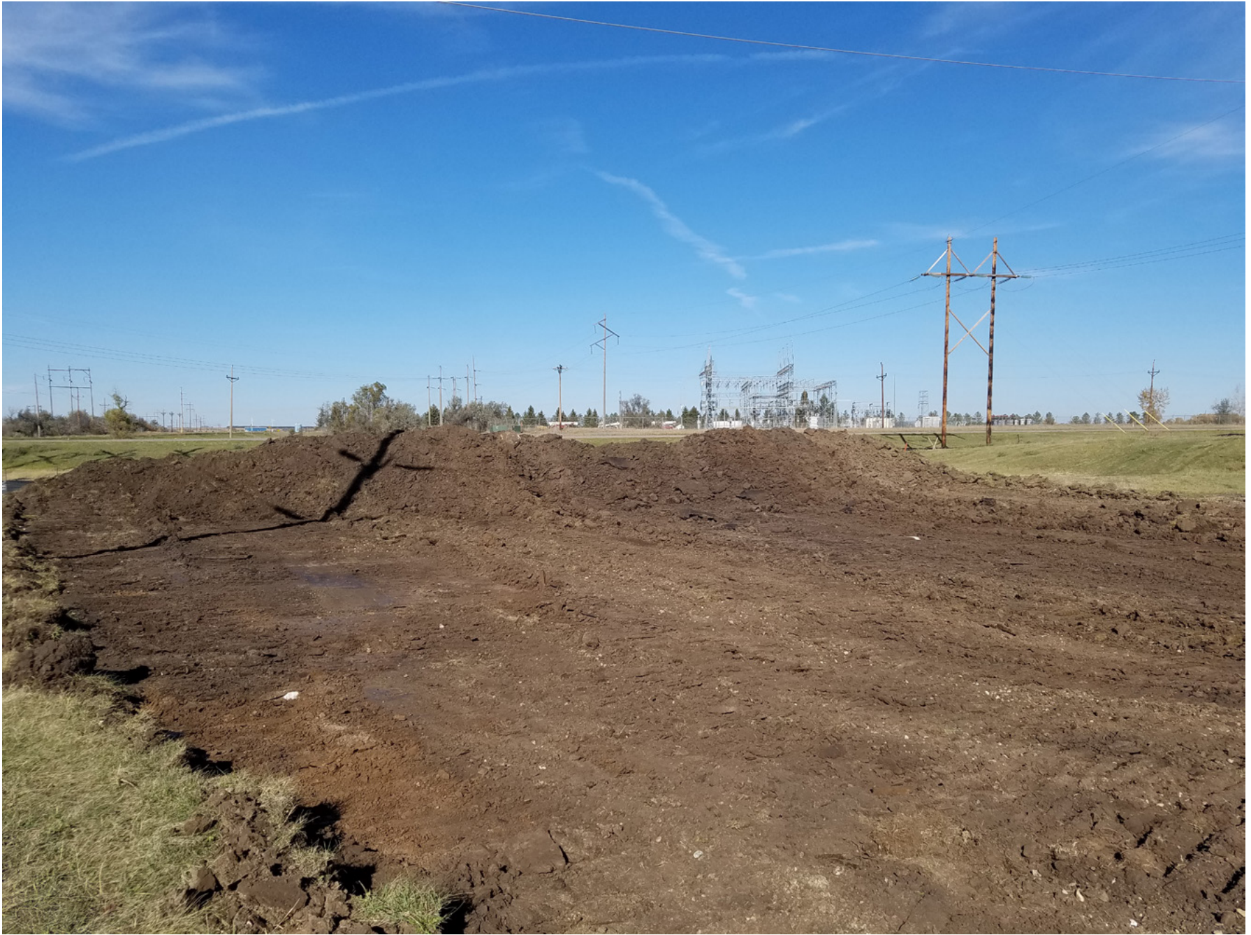
Photo 8 - Topsoil stockpile on north edge of the site looking north
