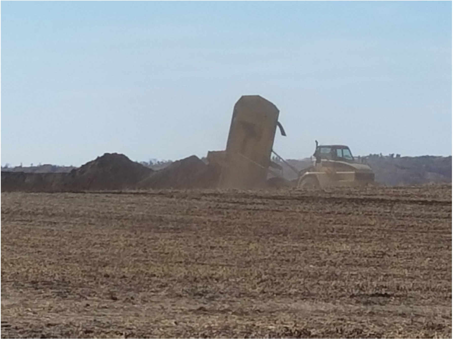
Photo 16 - Topsoil stockpile at southwest corner of site looking southwest
