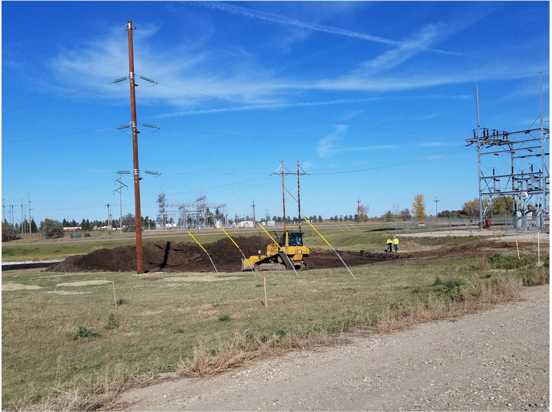
Photo 9 - Topsoil removal process on north side of approach looking northeast
