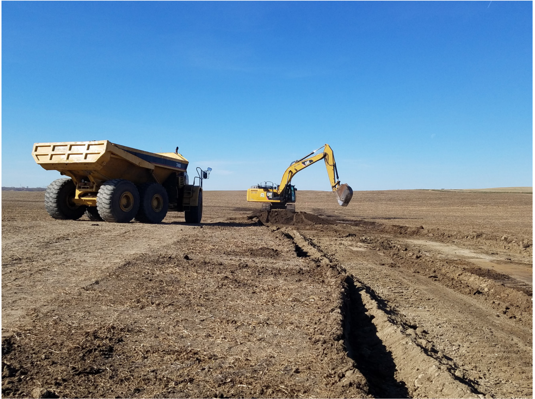
Photo 13 - Topsoil removal process looking west along north edge of pad
