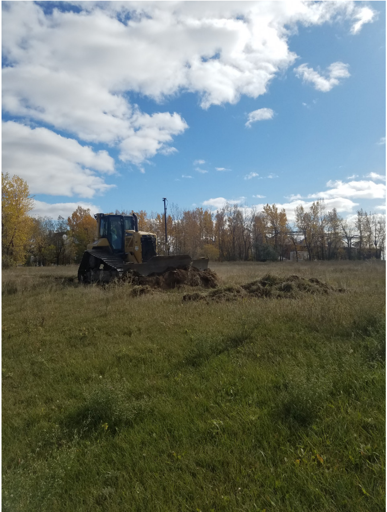
Photo 1 - Topsoil removal process
