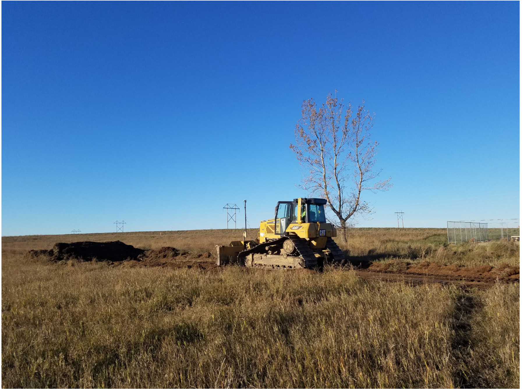
Photo 4 - Topsoil removal process looking at southwest corner of site
