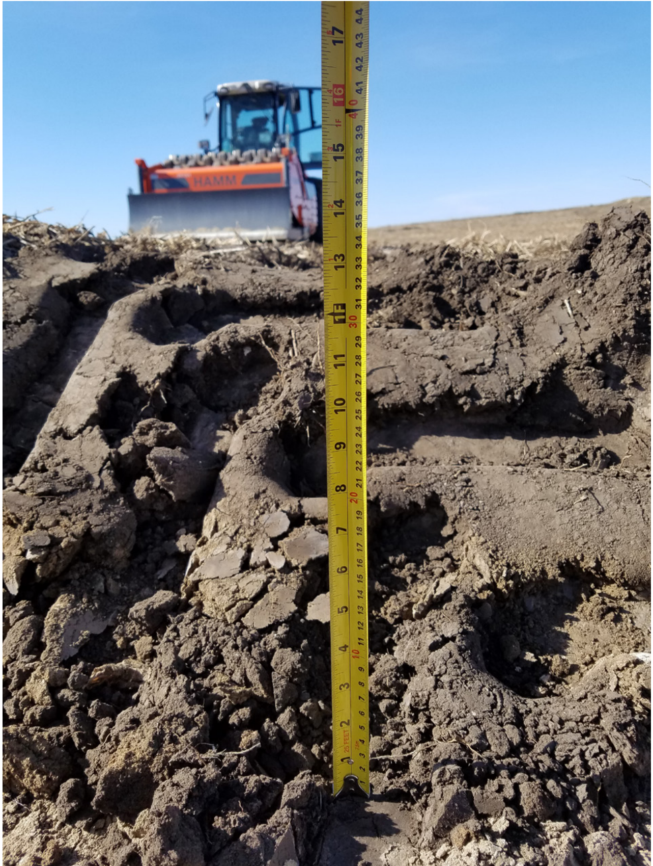
Photo 11 - 12" topsoil depth on access road looking west
