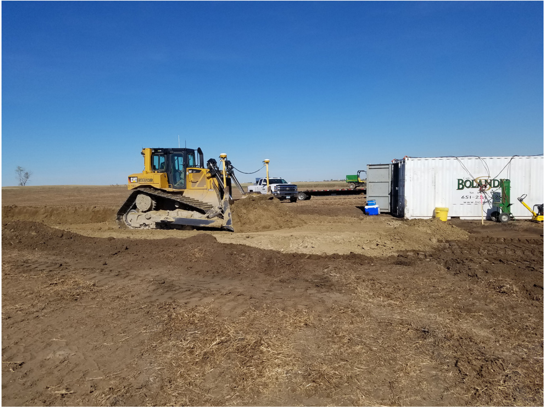
Photo 12 - Topsoil removal process at northeast corner of pad looking north
