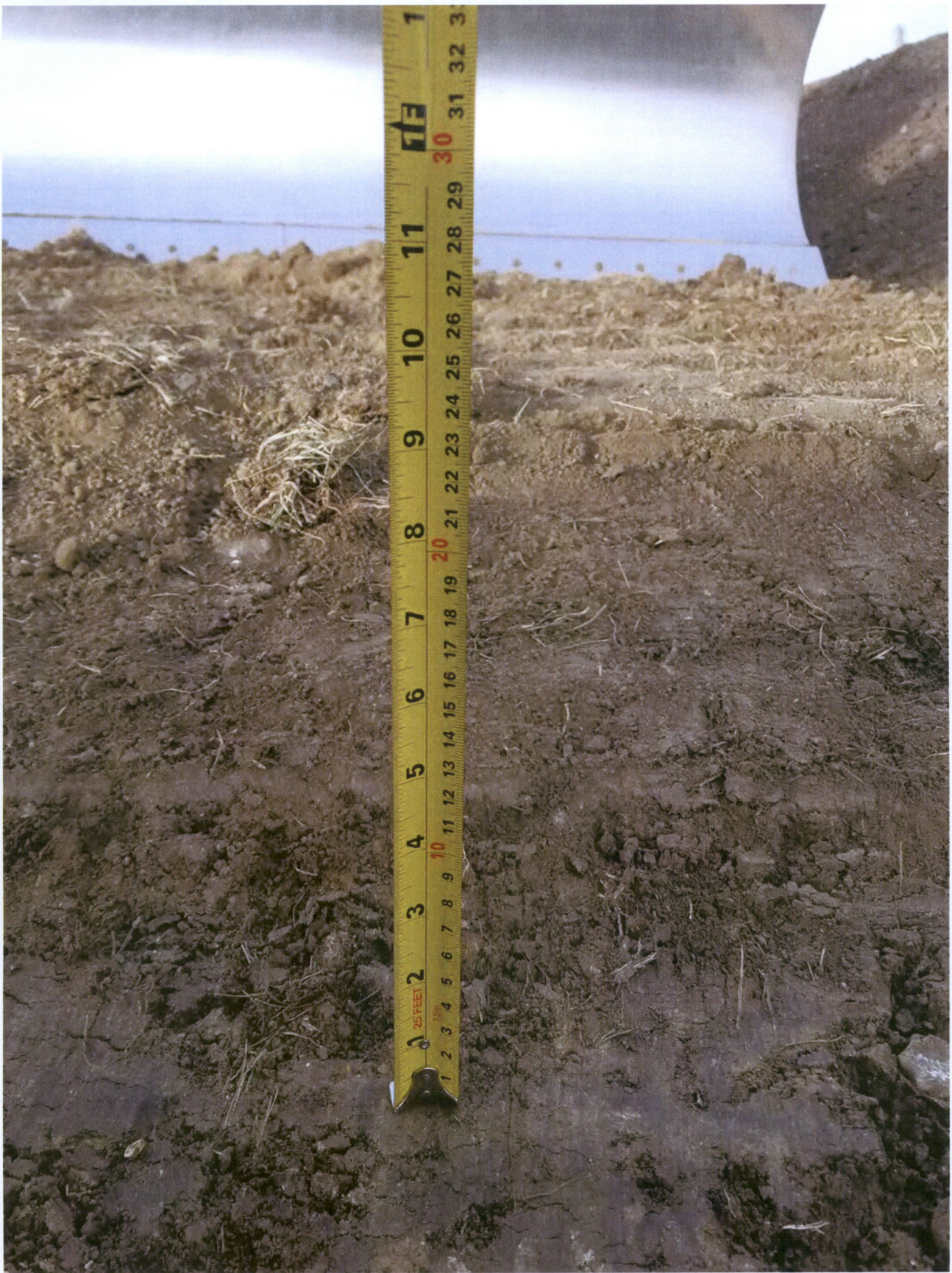
Photo 6 - 7" topsoil replacement depth northwest corner of site
