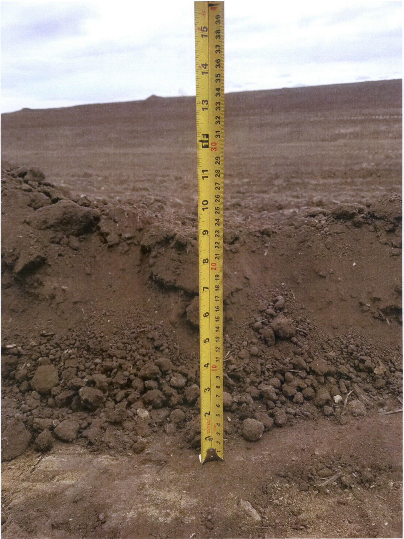
Photo 4 – 8" topsoil replacement depth on south bank of south pond
