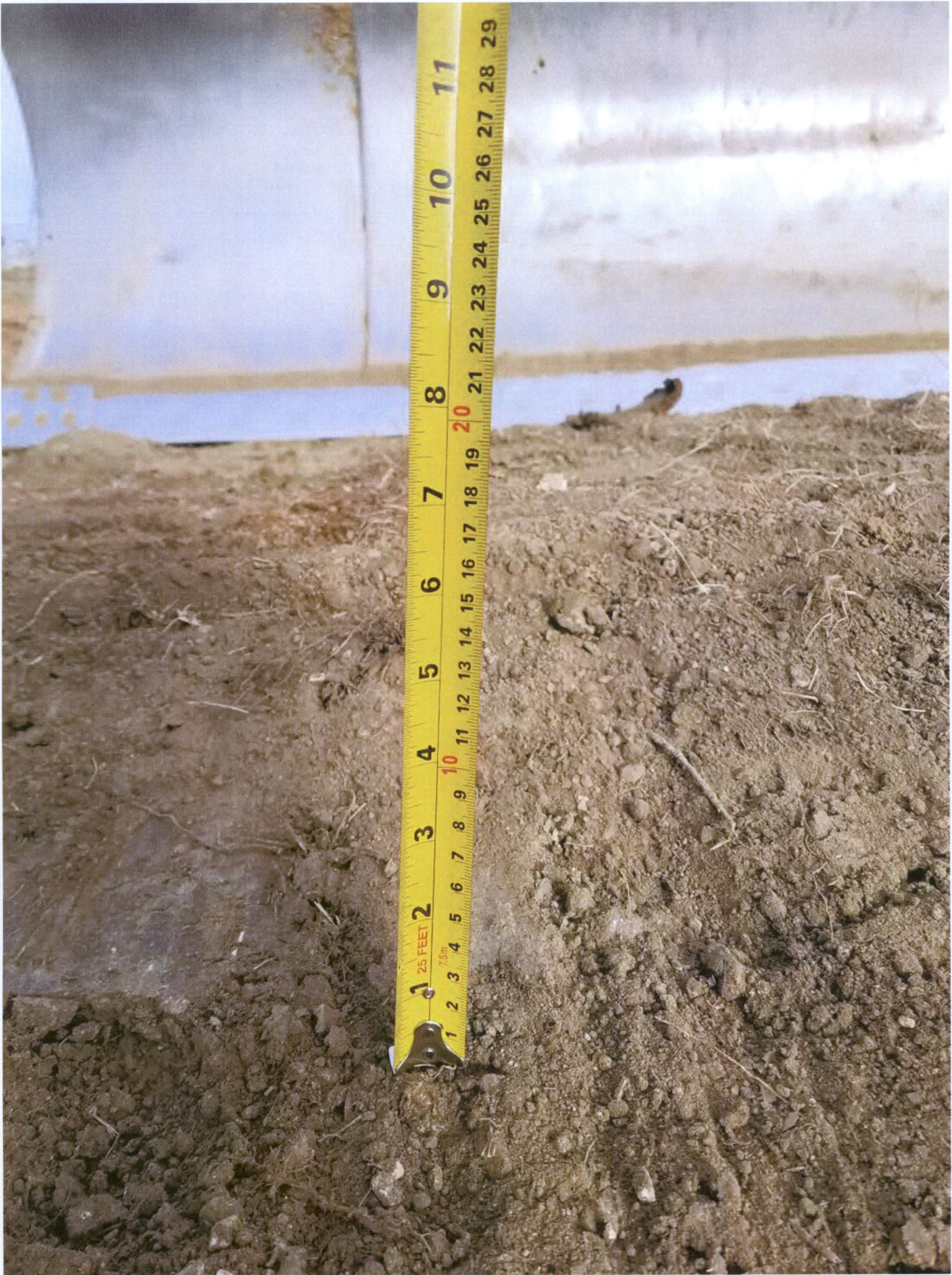
Photo 7 – 5" topsoil replacement depth southeast corner of site
