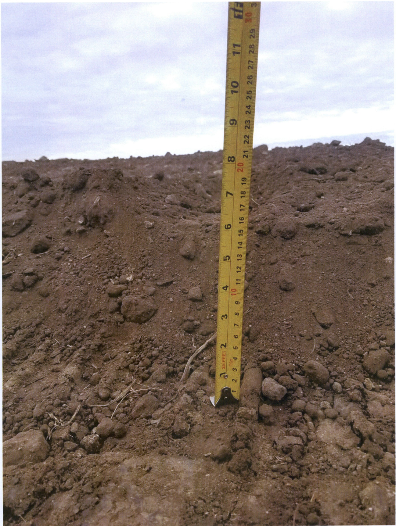
Photo 3 - 7" topsoil replacement depth on southwest bank corner of south pond
