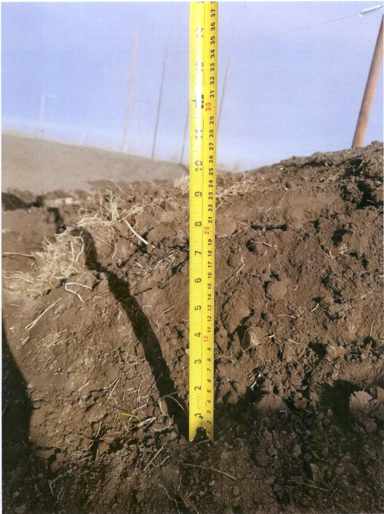
Photo 4 – 7" topsoil replacement depth northwest corner of site
