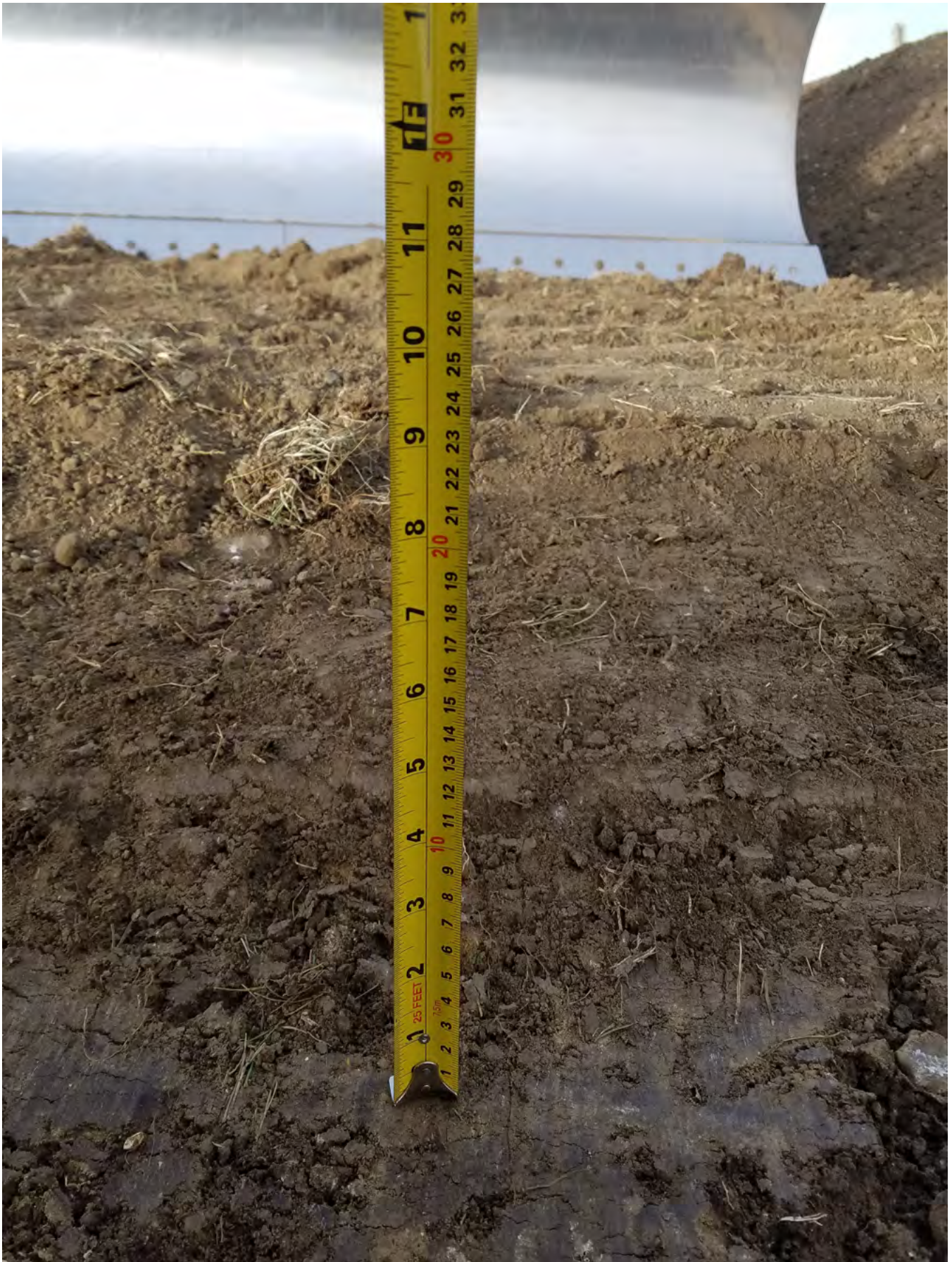
Photo 9 - 7" topsoil replacement depth northwest corner of site
