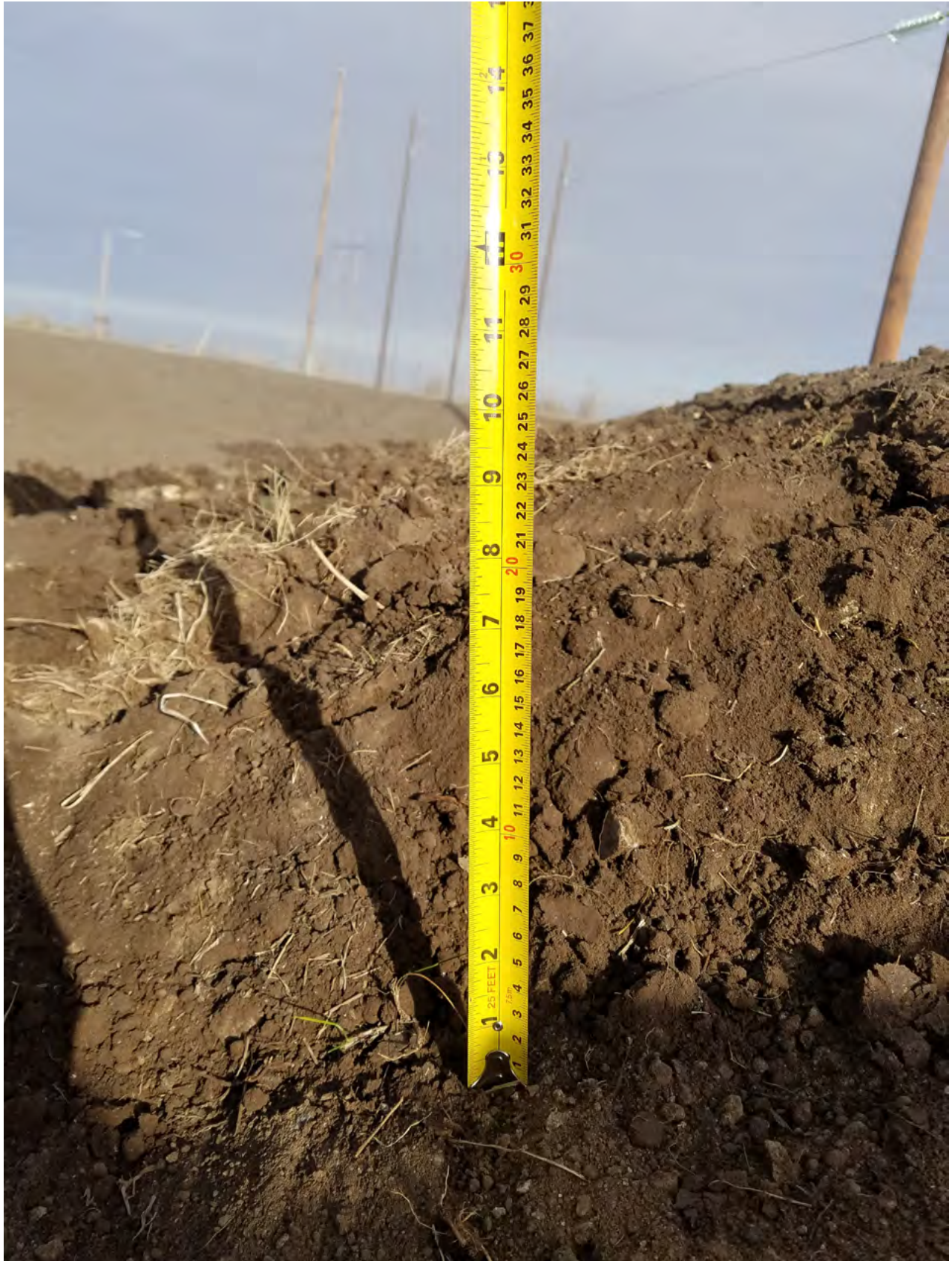
Photo 7 – 7" topsoil replacement depth northwest corner of site
