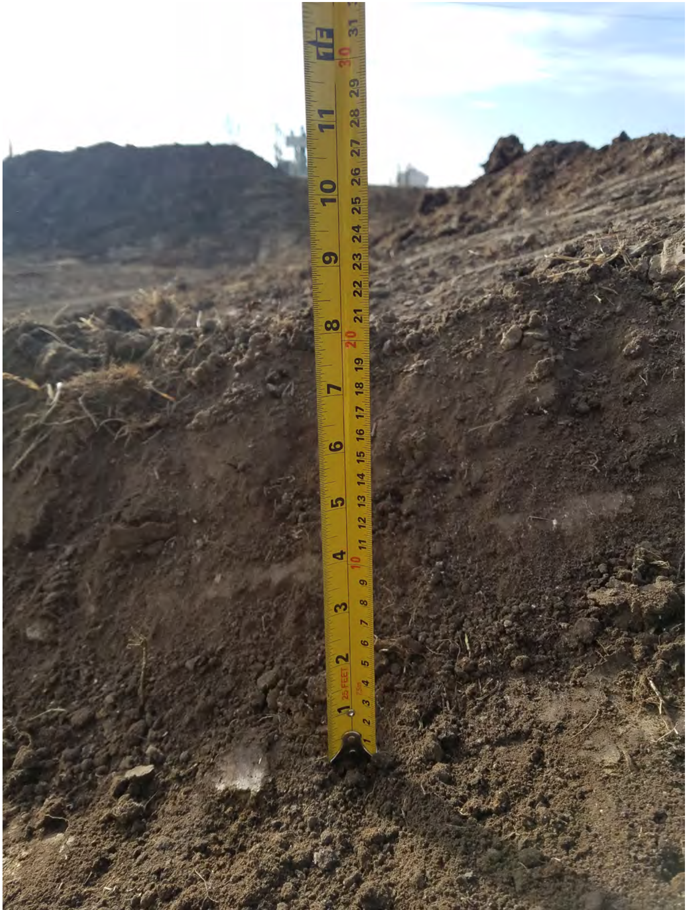
Photo 8 – 7" topsoil replacement depth northwest corner of site
