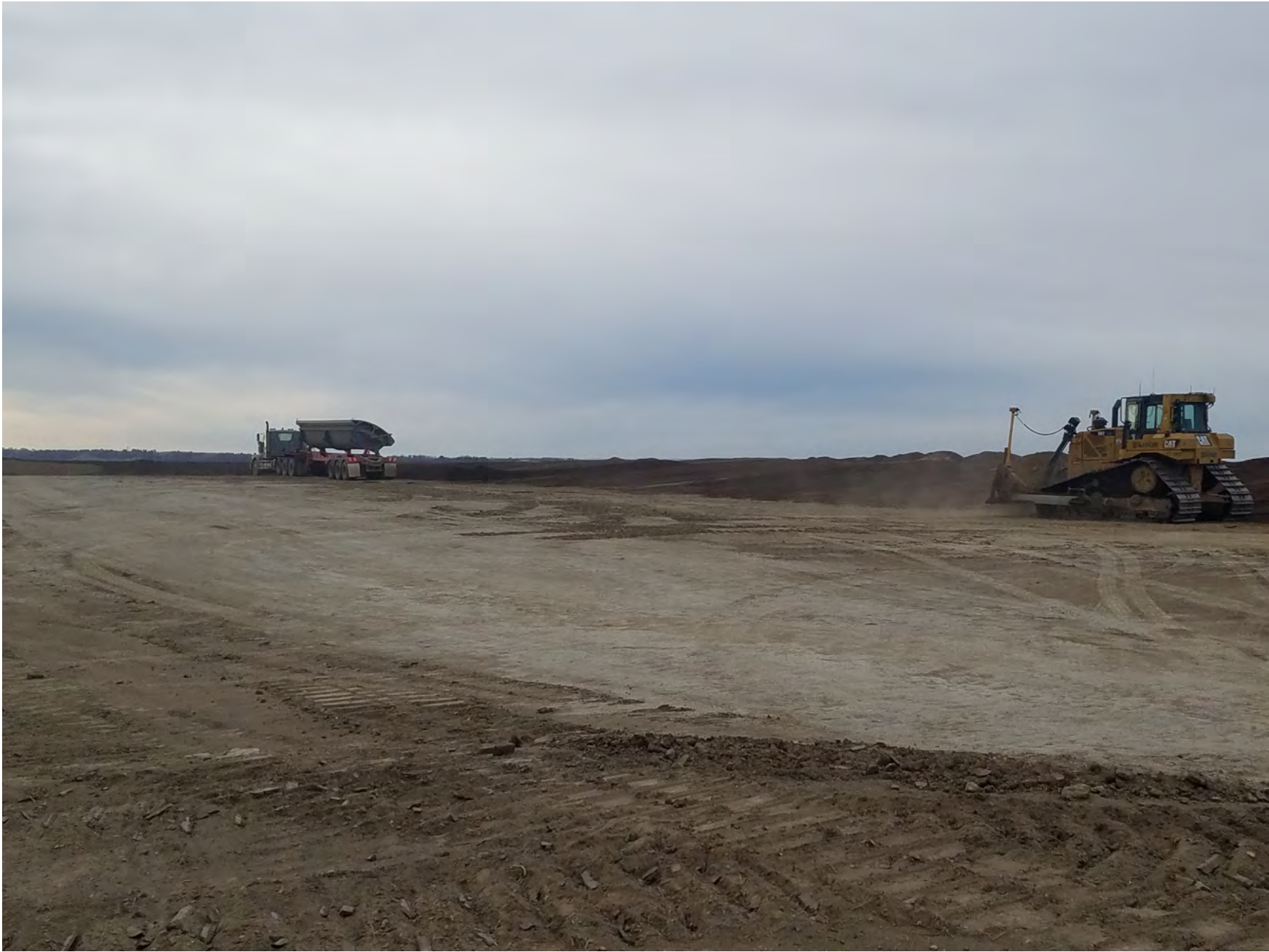
Photo 5 - Construction activity on site
