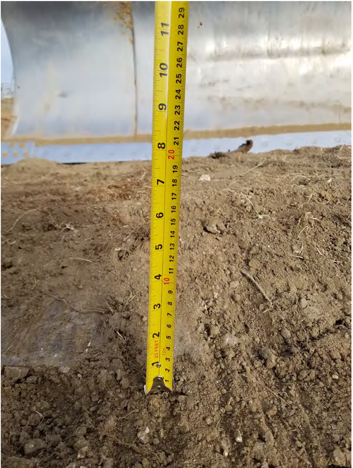
Photo 10 – 5" topsoil replacement depth southeast corner of site
