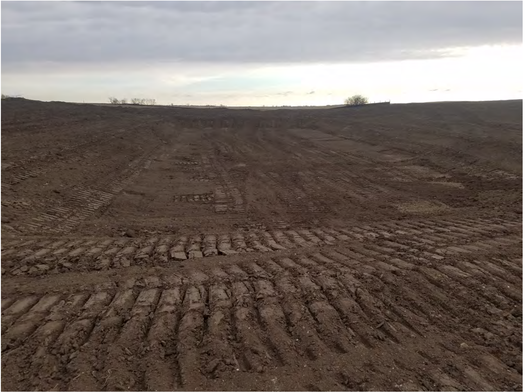
Photo 2 – Graded south pond with topsoil replacement
