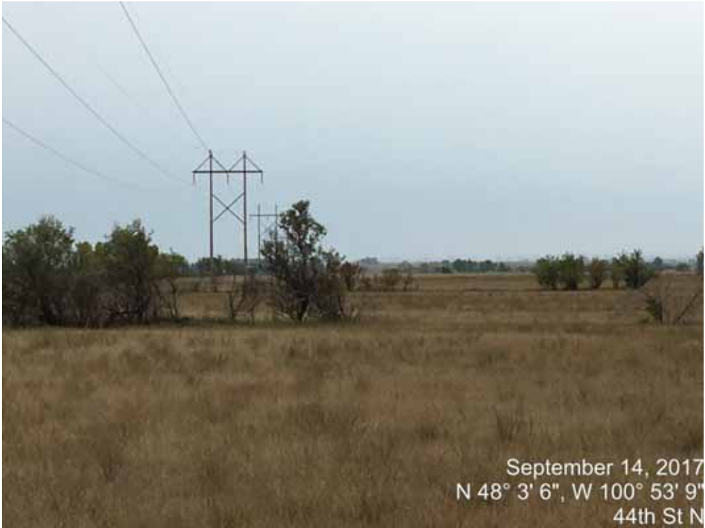
Photo 17 - Plot 10 and 11 overview from the road right of way
