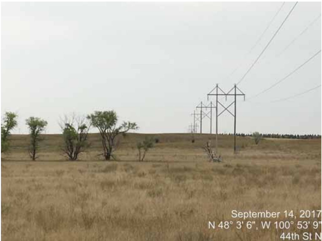
Photo 18 - Plot 12-14 overview taken from road right of way.
