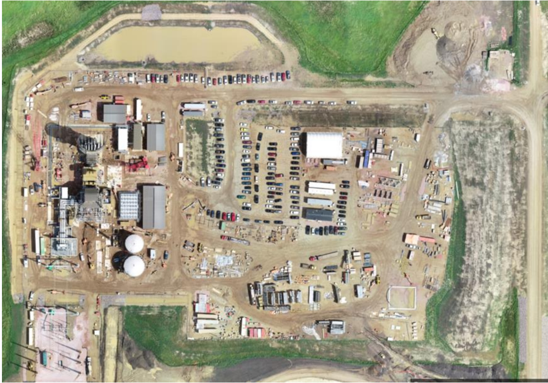
Site activity near beginning of quarter 7/1/2020
