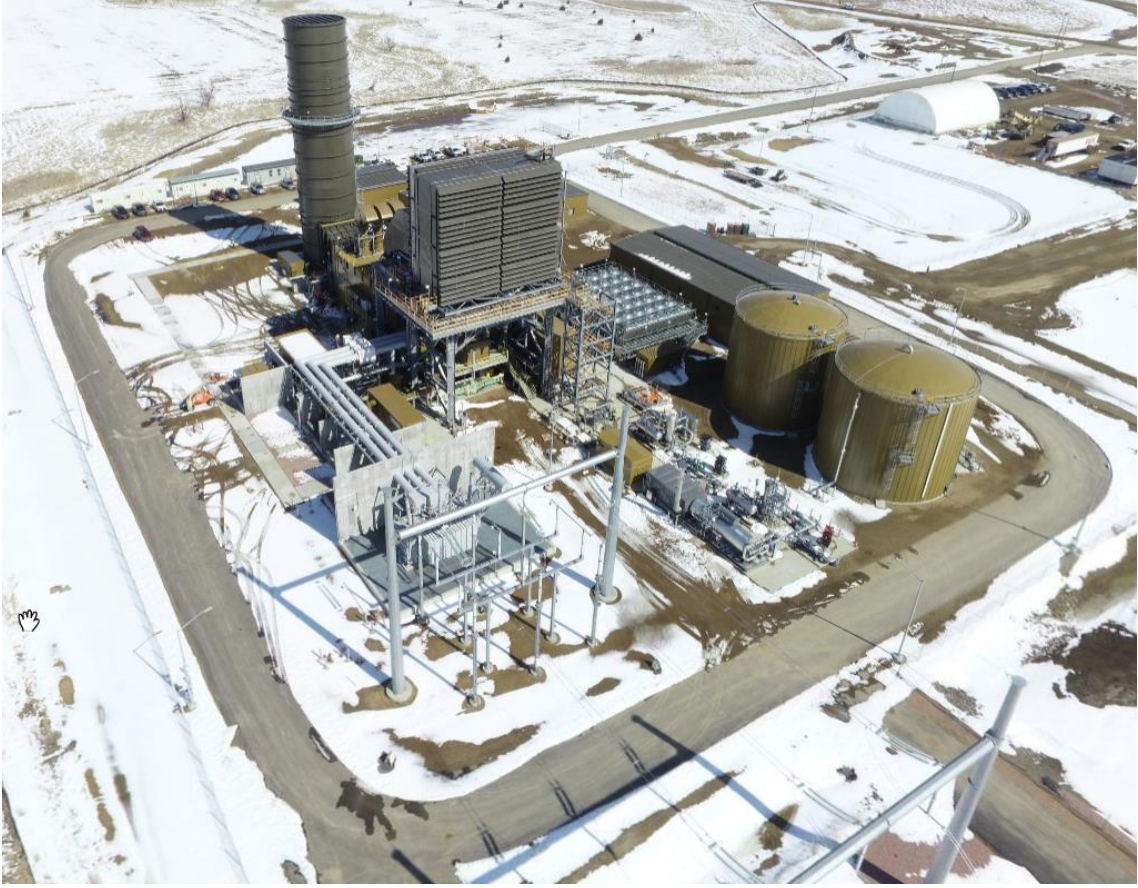
Astoria Station Aerial Photo
