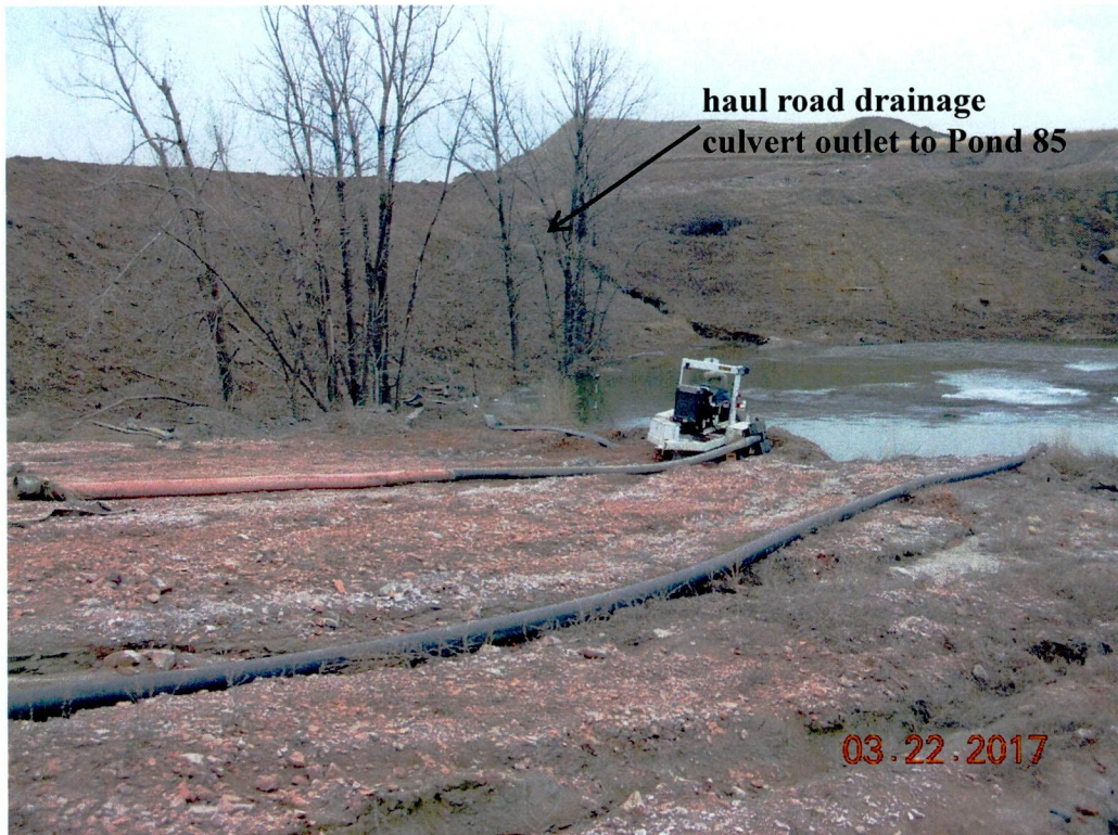
Figure 11. Haul road drainage culvert outlet to Pond 85 - see Figure 9 for location.
