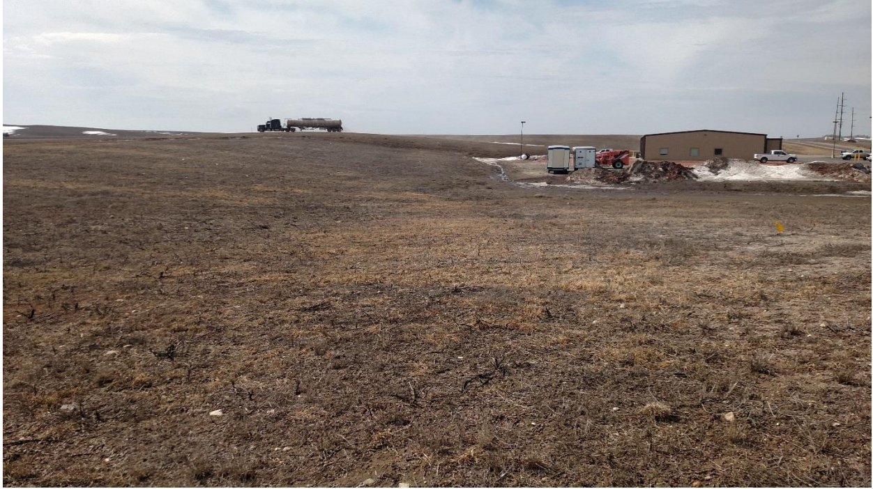
Photo 1. Gas plant expansion area facing west.
