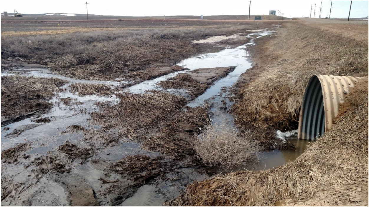
Photo 5. Ditch running west to east bordering northern edge of Survey Area.
