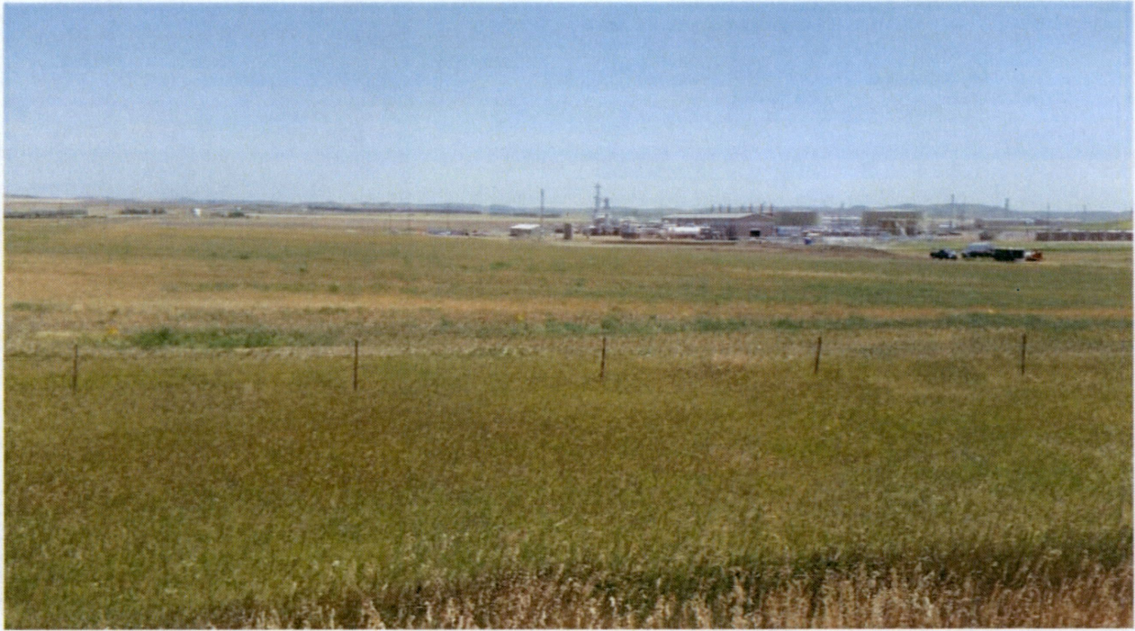
Figure 5. View from the western edge of the construction site looking east at the existing gas plant.
