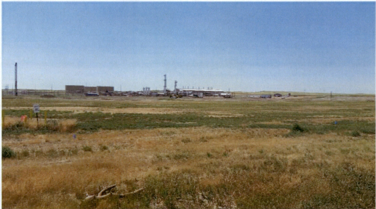
Figure 3. View from the northwest corner of the construction site looking southeast. Existing gas plant center of photo.
