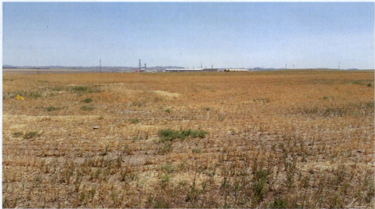
Figure 4. View from the northeast corner of the construction site looking southwest. Existing gas plant center of photo.
