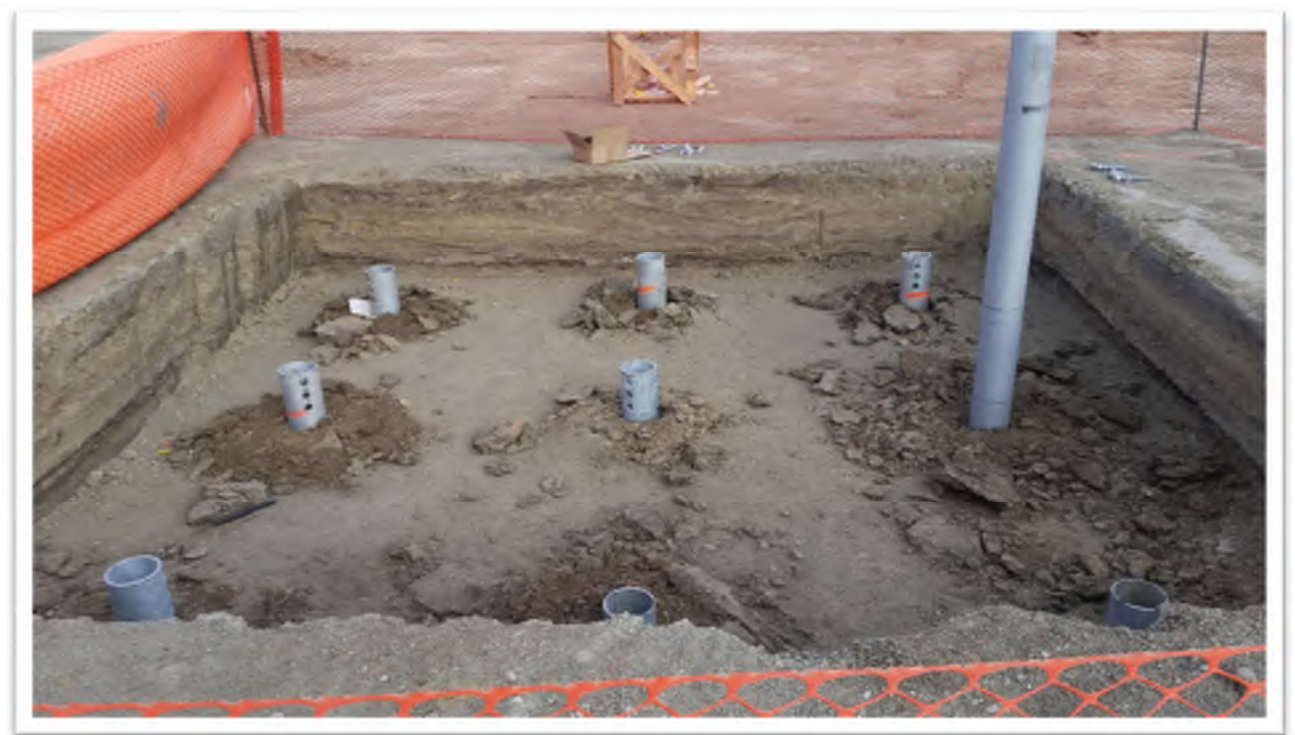
Figure 4. View of equipment foundation preparation.
