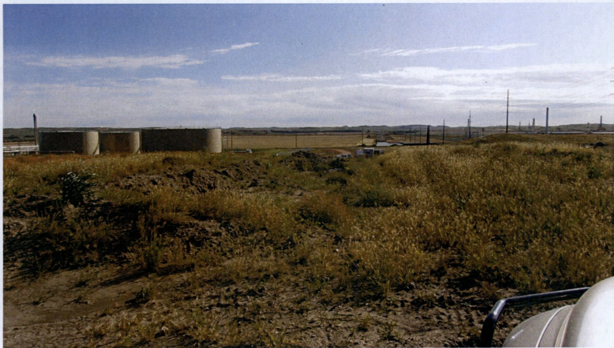
Figure 9. View of the truck turn around area that has seen limited reclamation.
