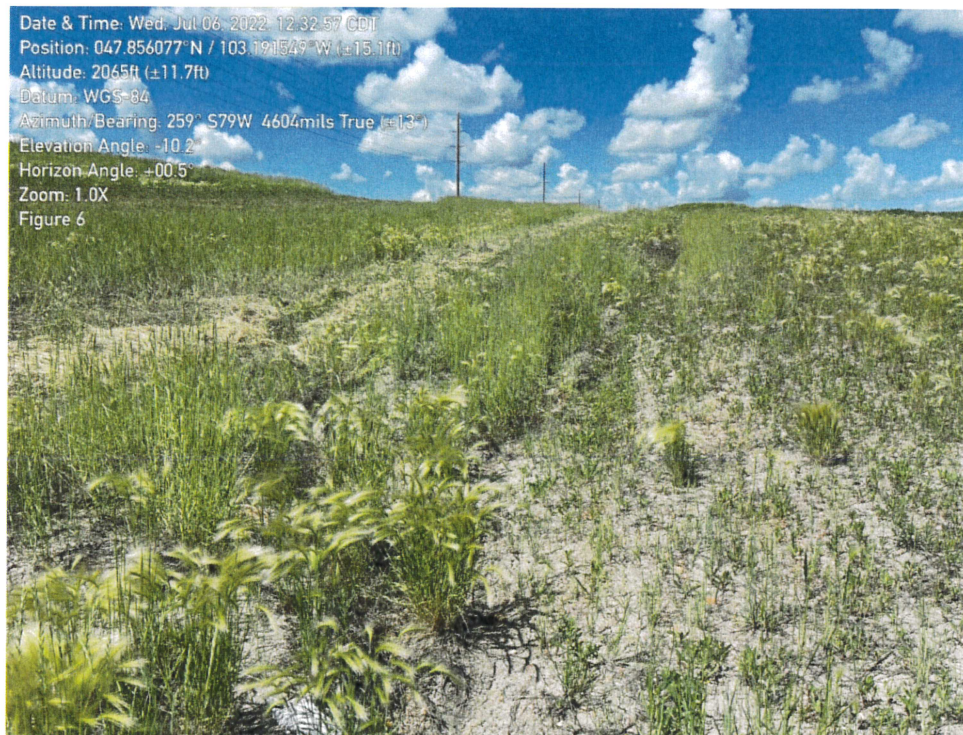
Figure 6: Minor rill erosion remains; however, vegetative cover has stabilized the soil.
