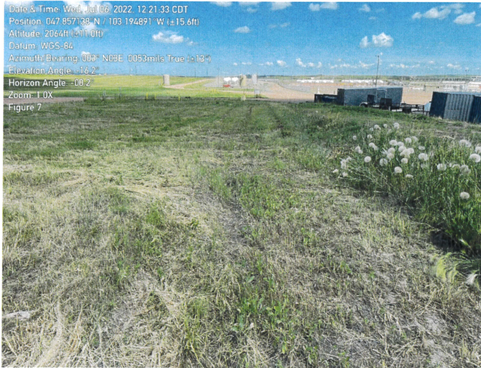
Figure 7: Erosion minimal and soil is stabilized.
