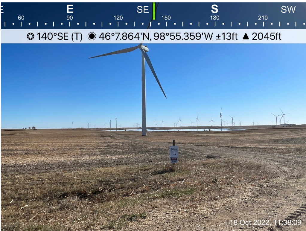
Report Photo #2: Access Road through Cropland and Turbine Site T-7
