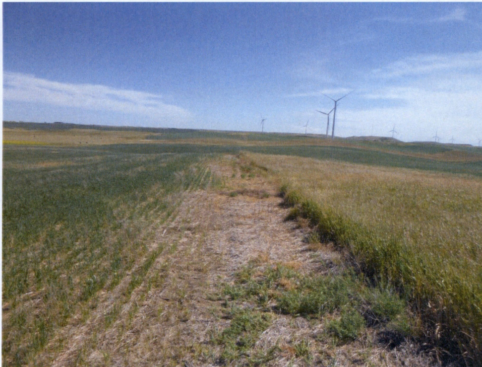
Photograph 2 (South): A view of proposed service road to the North Radar Tower location from the southwest corner of the proposed North Radar Tower staging area.
