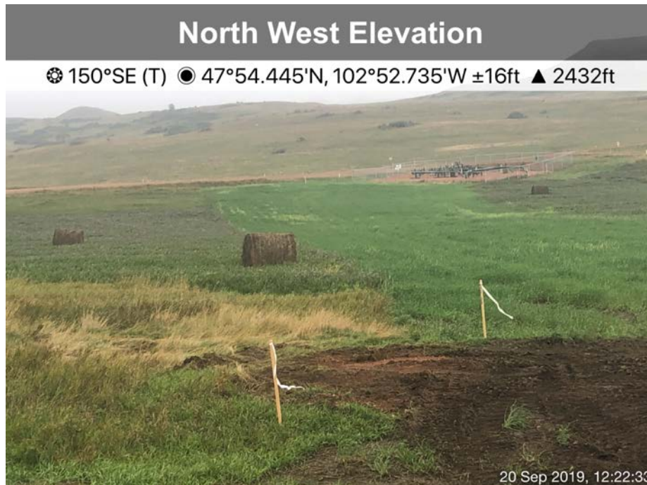
Photo 3 – Above Ground Piping near Pump Station
