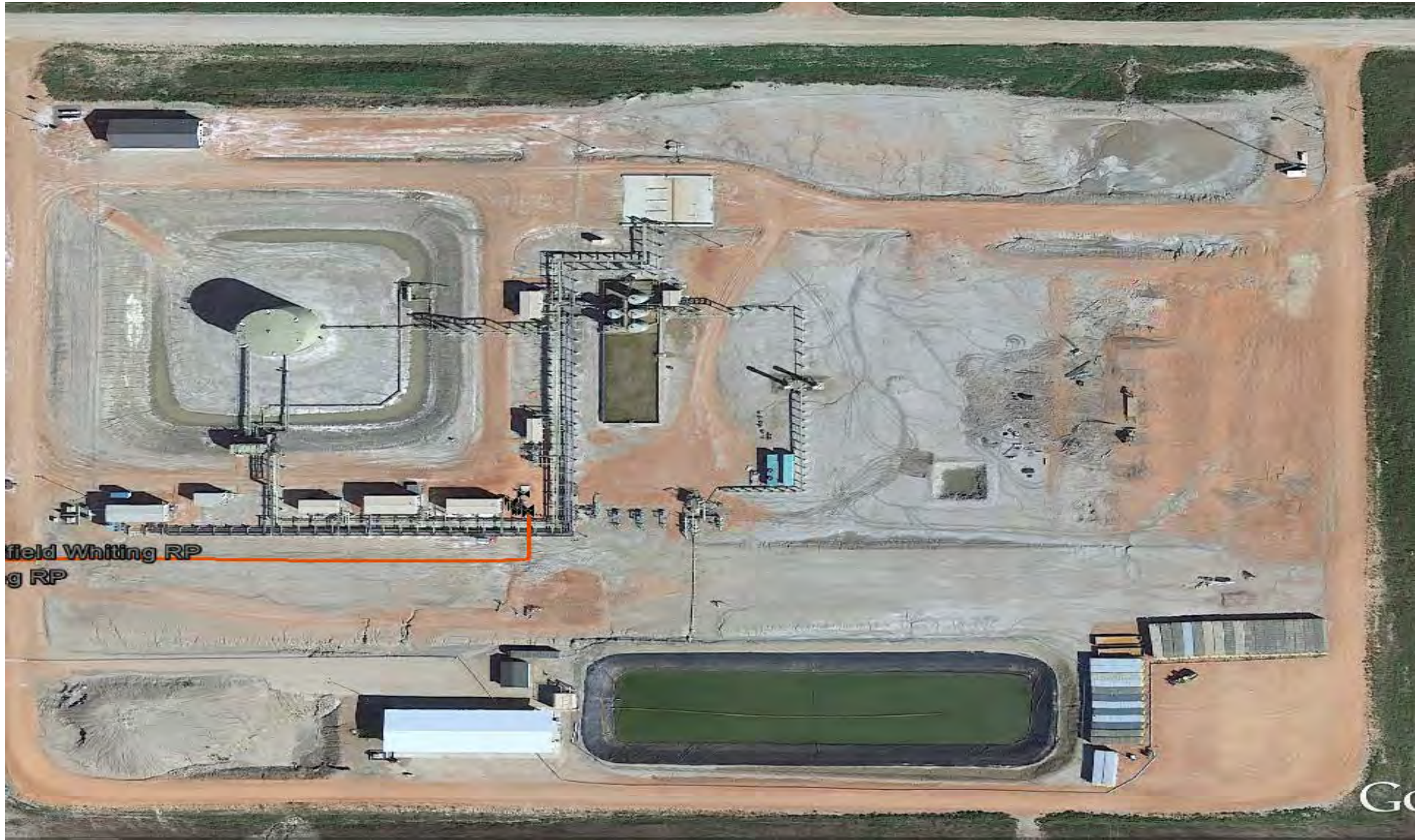
Figure J-31 Belfield Oil Terminal
