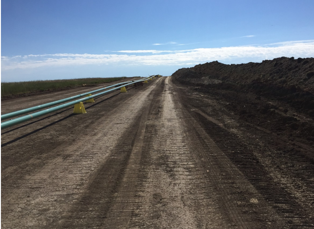
Photo 9. Facing: East. Location: 46.85963, -103.22839. Closer view of subsoil and topsoil stockpiles.
