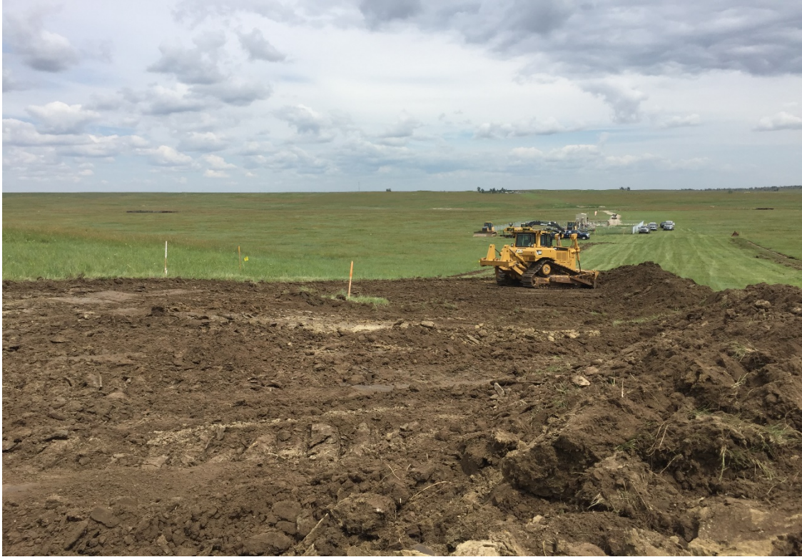
Photo 7. Facing: North. Location: 47.149667, -103.214934. Subsoil beginning to show at current grade. Depth of around 8 inches.
