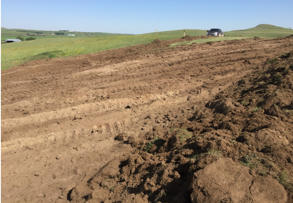
Photo 3. Facing: Northwest. Location: 47.80796, -103.17023. Topsoil stripped to depth of around 8 in. Subsoil reached with small amount of topsoil remaining will be leveled by final pass of grader.
