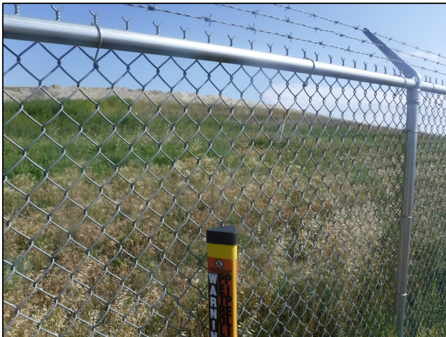
Photo 22. (Observation Point 12) Direction: Northeast. View of pipeline ROW from the Oasis Wild Basin natural gas processing plant at the southern-most point of the North Segment. Vegetation growth was 90%, though the co-native, weedy grass foxtail barley ( Hordeum jubatum ) was the dominant species. Soil was replaced to match topography. Note the chain link fence for public safety.
