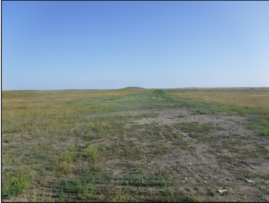
Photo 7. (Observation Point 5) Direction: North. View of reclaimed pipeline ROW through range/grazing land along the South Segment. Planted grasses were growing in this area at about 20% cover. Annual weed species dominated the reclaimed ROW at approximately 30-40% cover, with 50% bare ground. Further reclamation may be necessary in this area.
