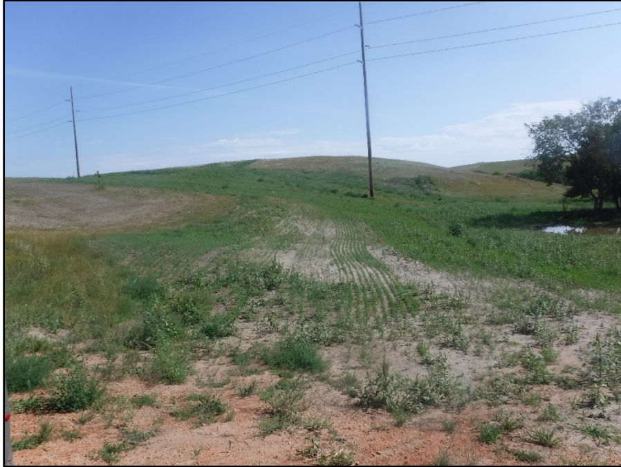
Photo 25. (Observation Point 14) Direction: Northeast. View of pipeline ROW along a slope on the Northern Segment. Vegetative growth was limited in this area, growing to about 40% cover with 60% bare ground. These conditions could make this hillslope susceptible to erosion. Note the woody draw on the right hand of the photo.
