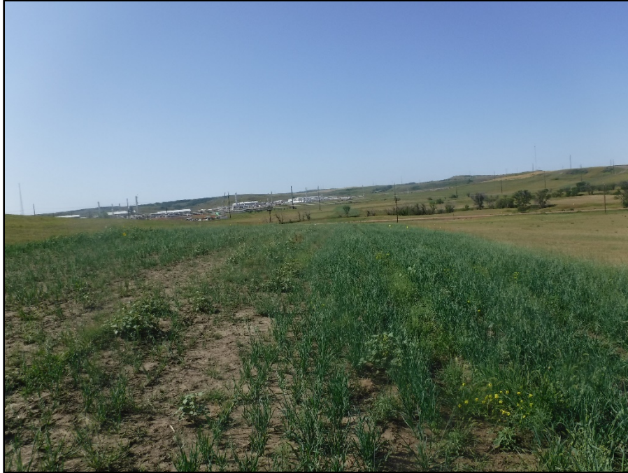
Photo 23. (Observation Point 13) Direction: Southwest. View of Pipeline ROW through rangeland on the North Segment. Vegetative growth was approximately 50-60% ground cover with minimal annual weeds. Dominant species included smooth brome, crested wheat grass, and oats.
