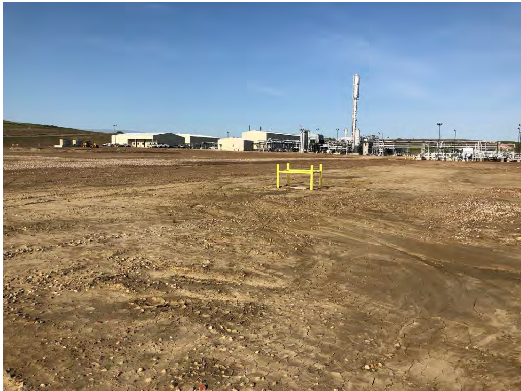
Photograph 6. View of the undeveloped eastern half of the Project Area, looking southwest.
