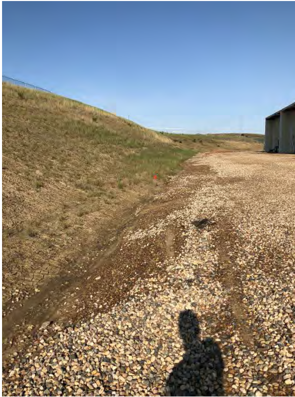
Photograph 1. View of the southern edge of the Project Area, facing west.
