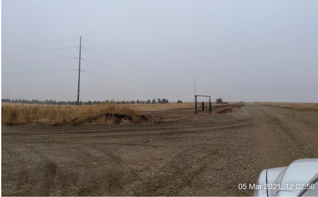
Photo #6: Transmission Line along 24 th Ave SE
