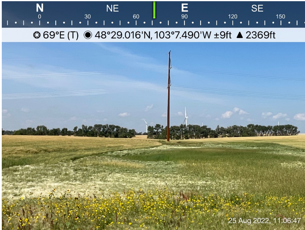
Report Photo #3: Transmission Pole near Wetland
