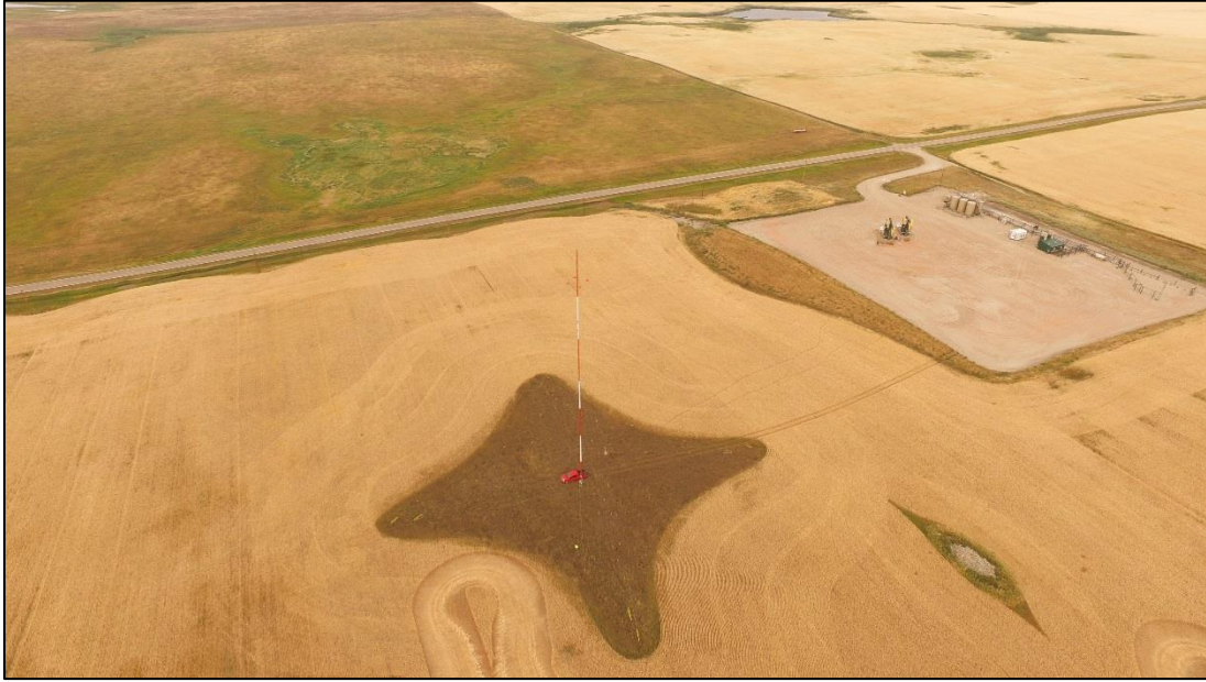
Photo 1: Tower 0262 and landscape. Photo taken with unmanned aerial system on August 16, 2018.
