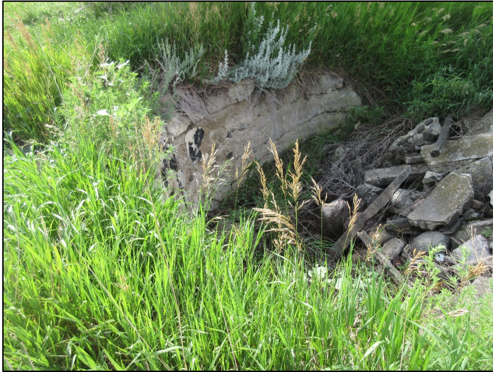
Photograph B-15: Partially collapsed and backfilled ice house, site A-102, facing southeast.
