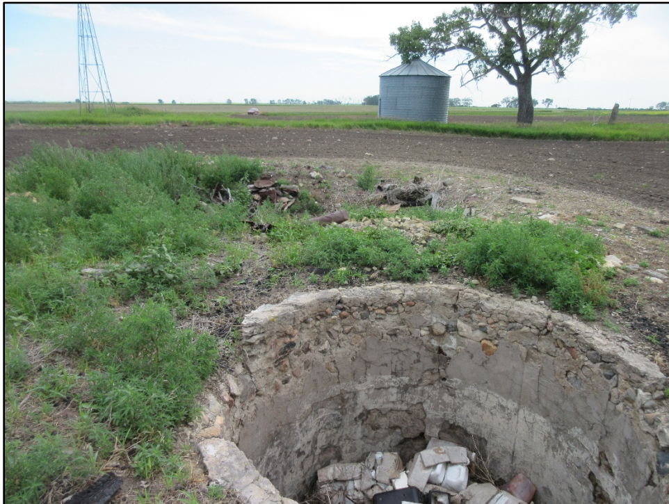
Photograph B-12: Cistern (foreground) and adjacent trash-filled basement, site A-102, facing east.
