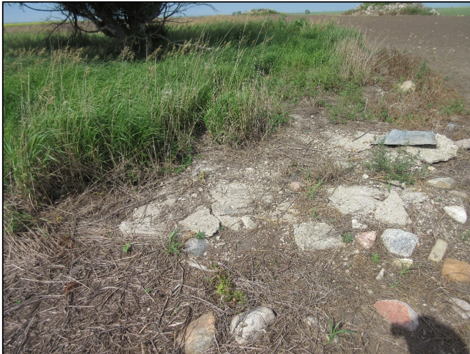
Photograph B-14: Remnant of concrete pad in northern portion of site A-10, facing north.
