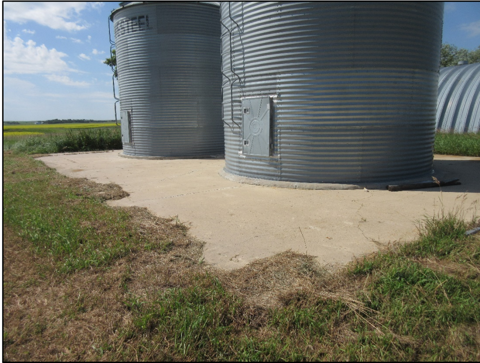
Photograph B-7: Modern grains bins on concrete pad barn floor, site A-101, facing northwest.
