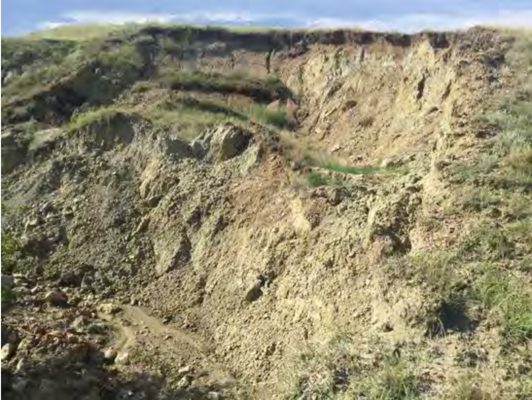
Photo Type: Slope movement evidence | Photo Bearing: 333 degrees Photo Description: Looking at scarp and slide mass.
