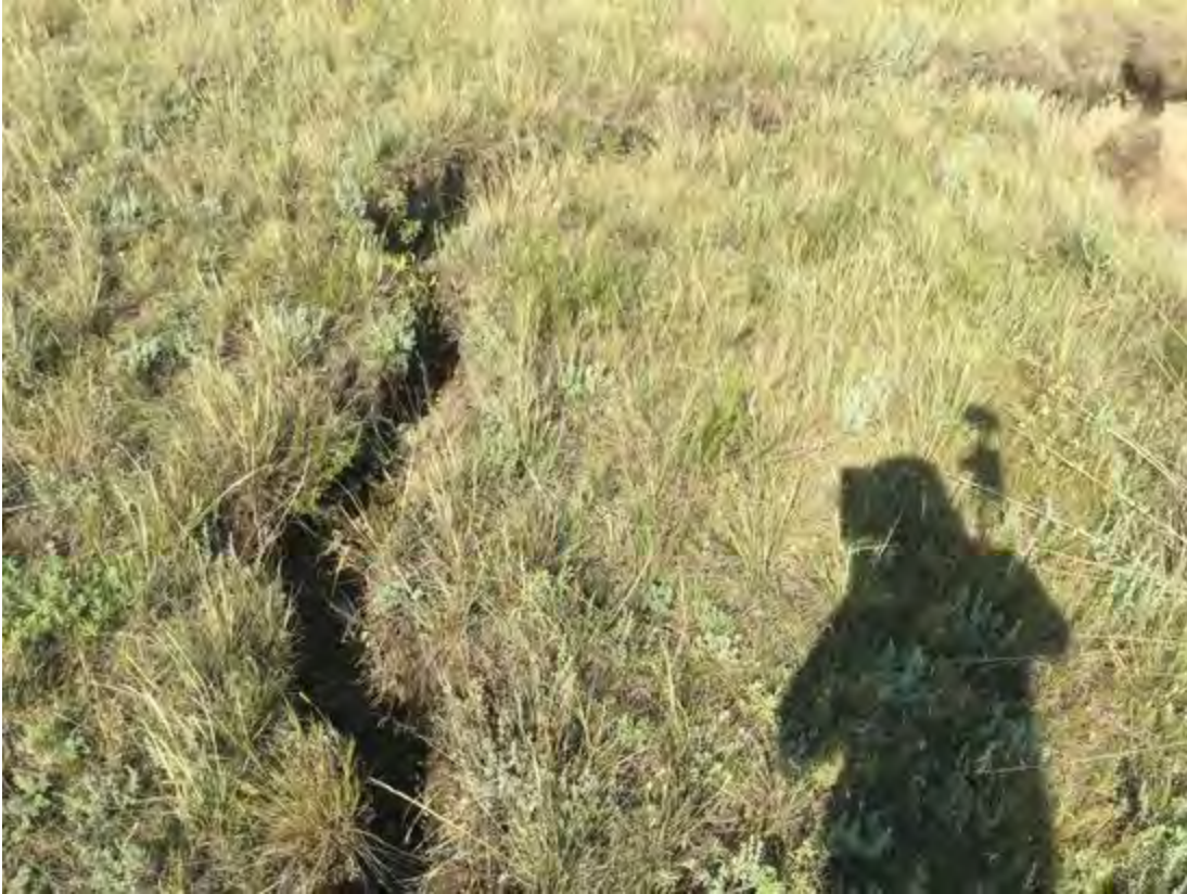
Photo Type: Slope movement evidence | Photo Bearing: 64 degrees Photo Description: Looking at tension crack.
