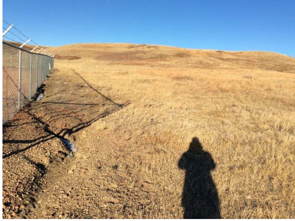
Photo 1: Pipeline start (Section 8, T147N, R101W)
