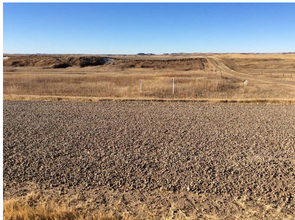
Photo 17: 138 th Avenue crossing.
