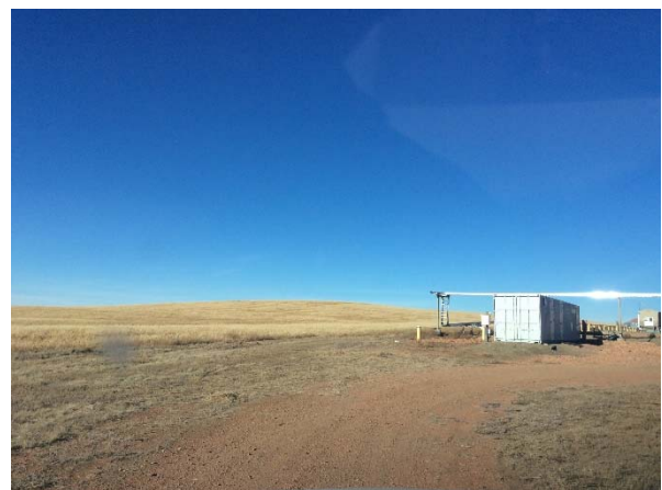
Photo 29: Terminal end of pipeline at Belle Fourche truck load out facility.
