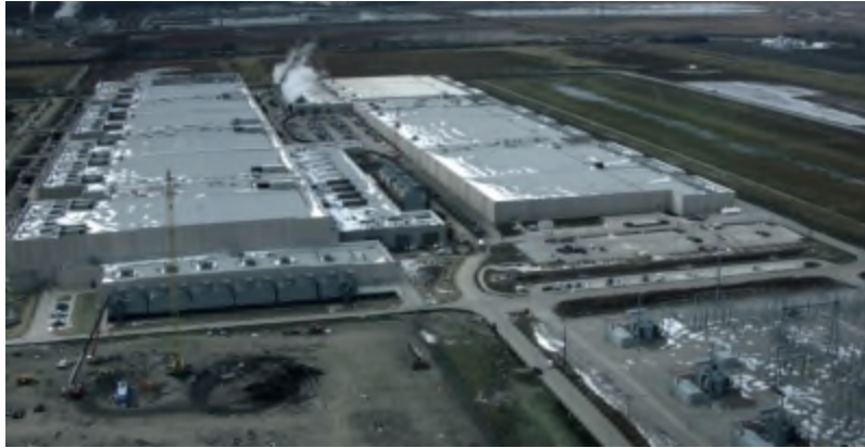
Figure 7 Aerial Photo 8 of Google Data Center Campus in Council Bluffs, Iowa
