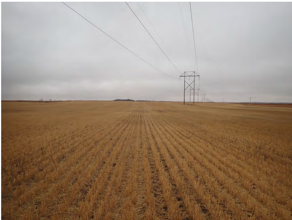
Figure 16. Overview of the survey area substation. View to the northeast.
