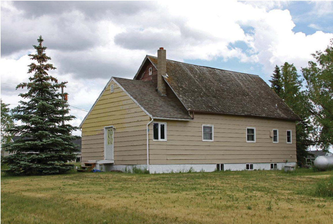
Figure 19. Site 32ML947 ineligible residence, June 18, 2019, looking southeast (IMG_2533.jpg).
