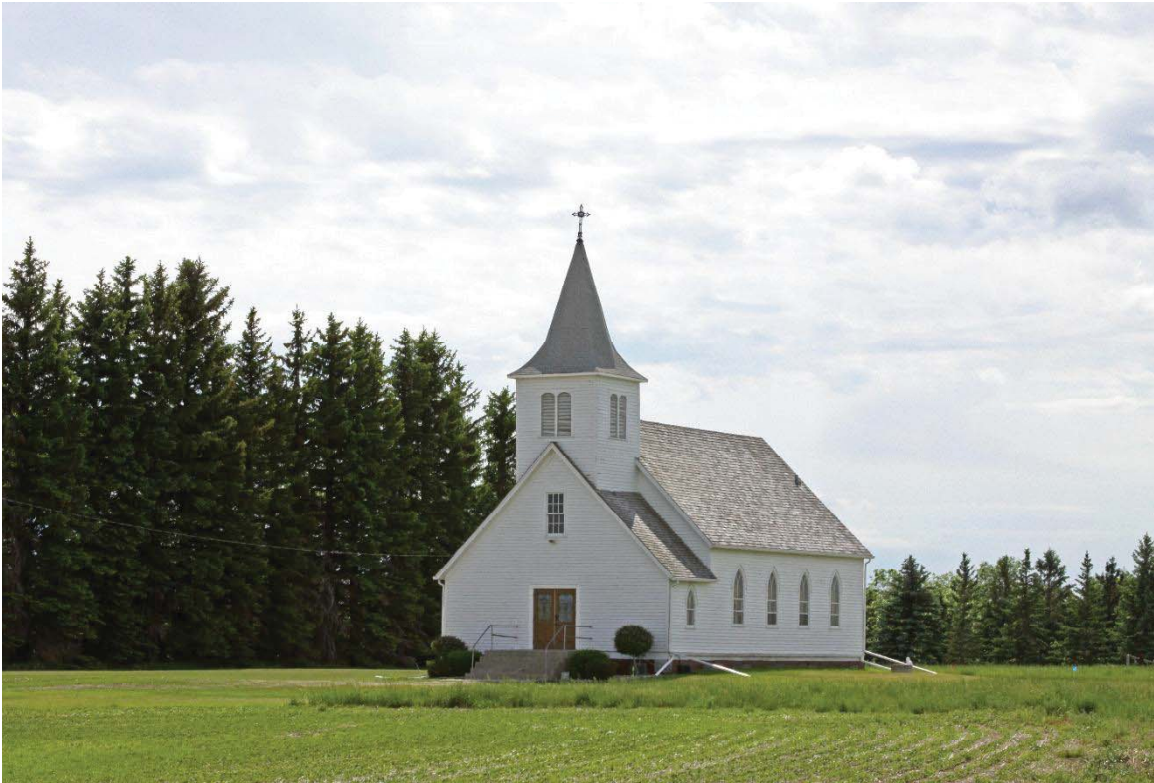
Figure 10. Site 32WD1590 church, June 14, 2019, looking southwest (IMG_2169.jpg).
