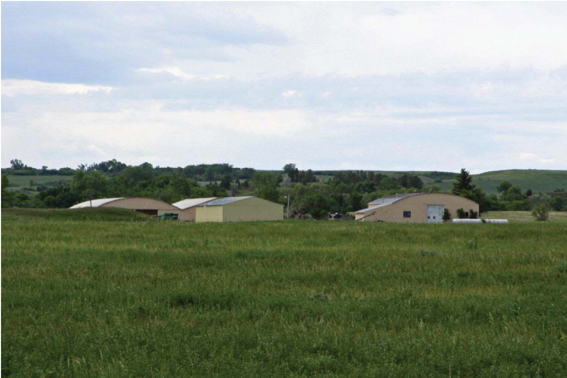
Figure 7. Site 32WD2462, June 14, 2019, looking south (crop of IMG_1993.jpg).
