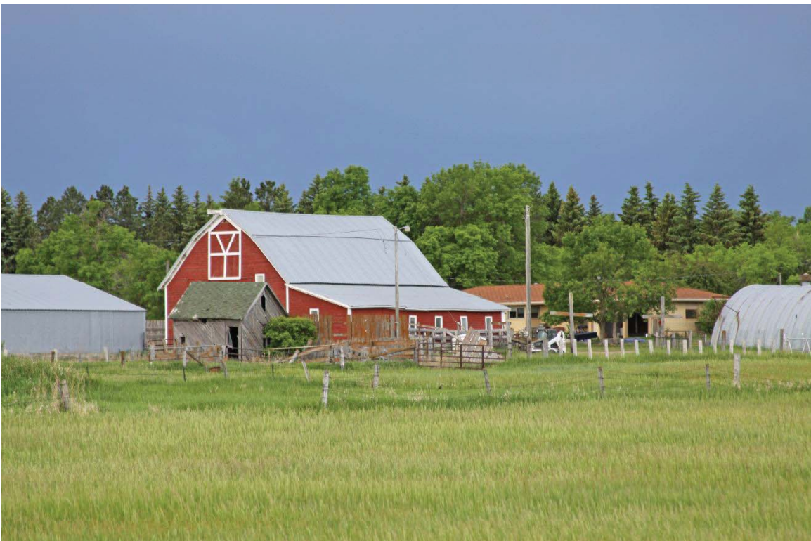
Figure 3. Site 32MH474, June 14, 2019, from 35th St N facing southwest (IMG_1832.jpg), with focus on the gambrel roof dairy barn. The storehouse is in the foreground.
