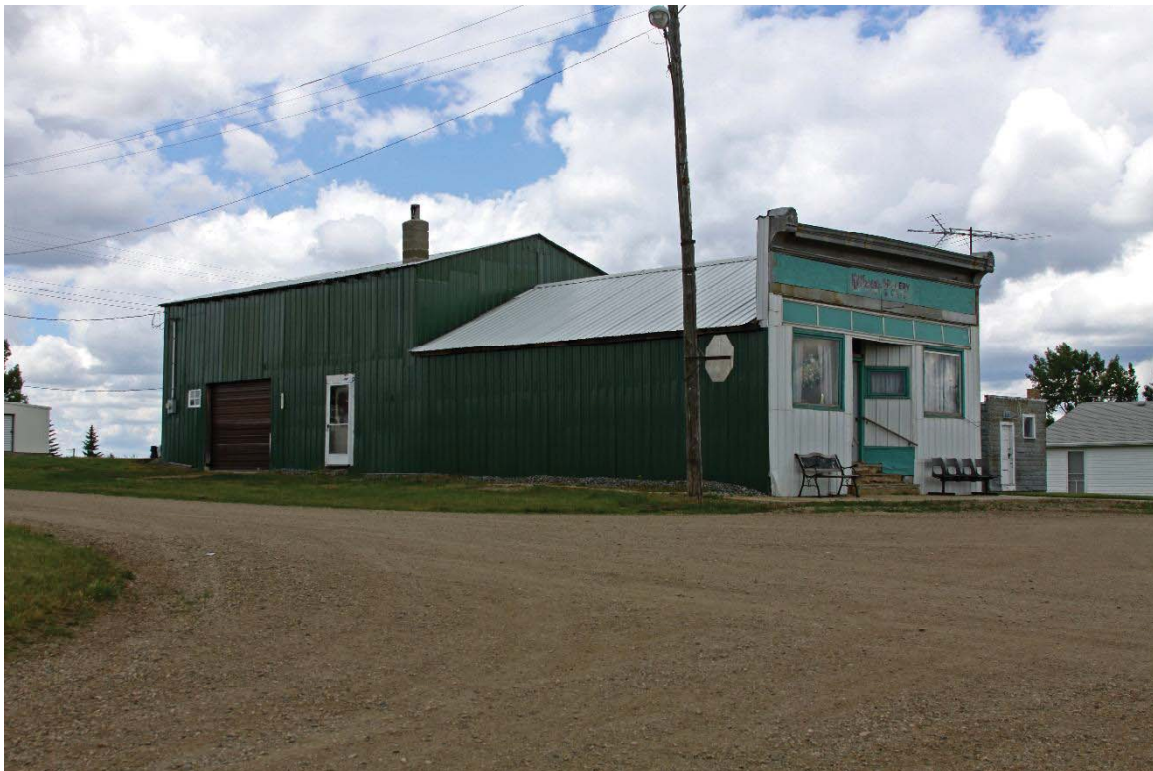
Figure 18. Site 32ML1363 Boomtown/False Front commercial building, June 18, 2019, looking northwest (IMG_2458.jpg).
