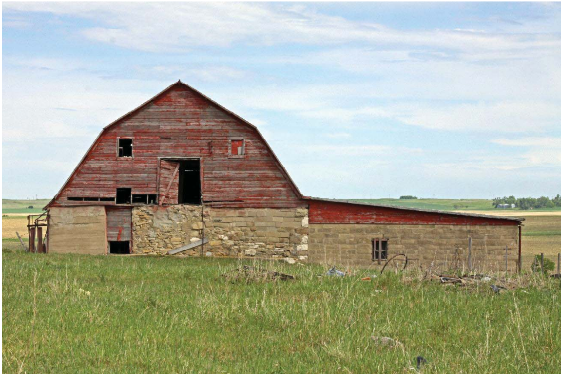
Figure 13. Site lead 32WDx747 gambrel barn, June 14, 2019, looking southeast (IMG_2178.jpg).
