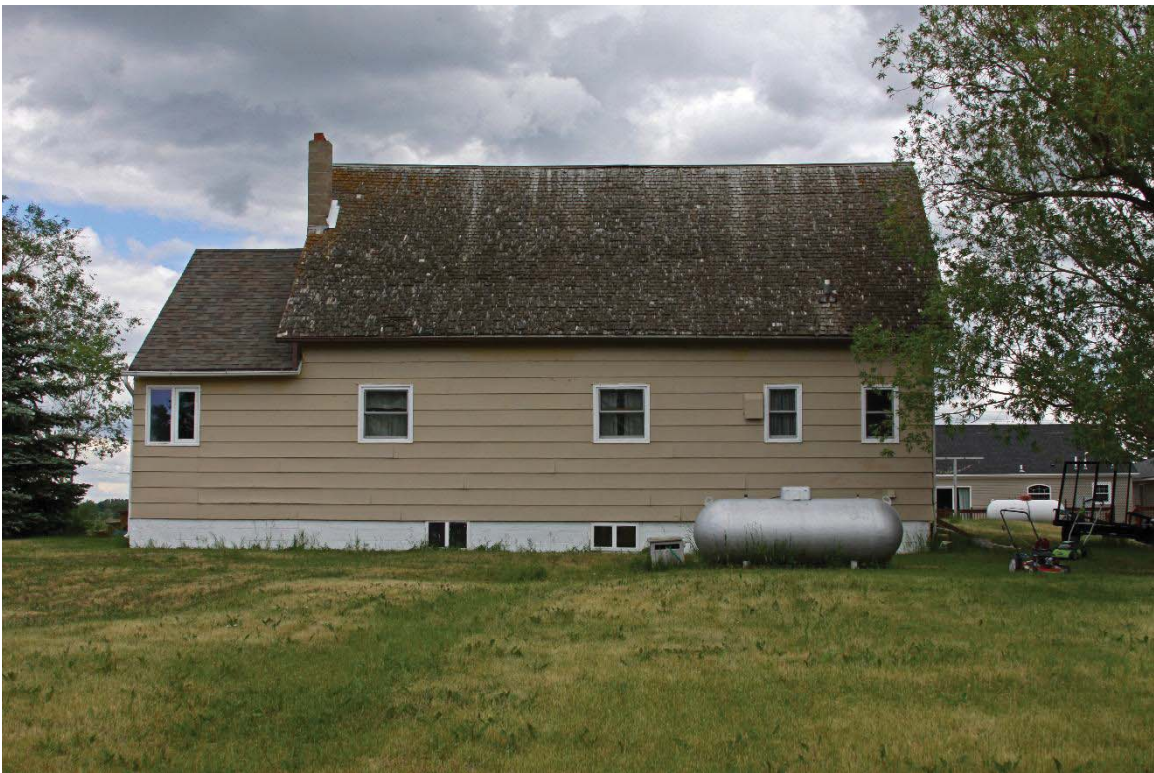
Figure 20. Site 32ML947 ineligible residence, June 18, 2019, looking east (IMG_2525.jpg).
