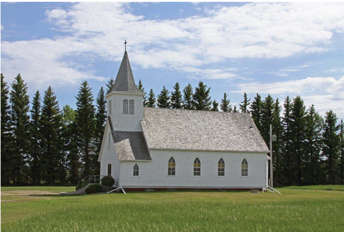
Figure 11. Site 32WD1590 church, June 14, 2019, looking south (IMG_2171.jpg).
