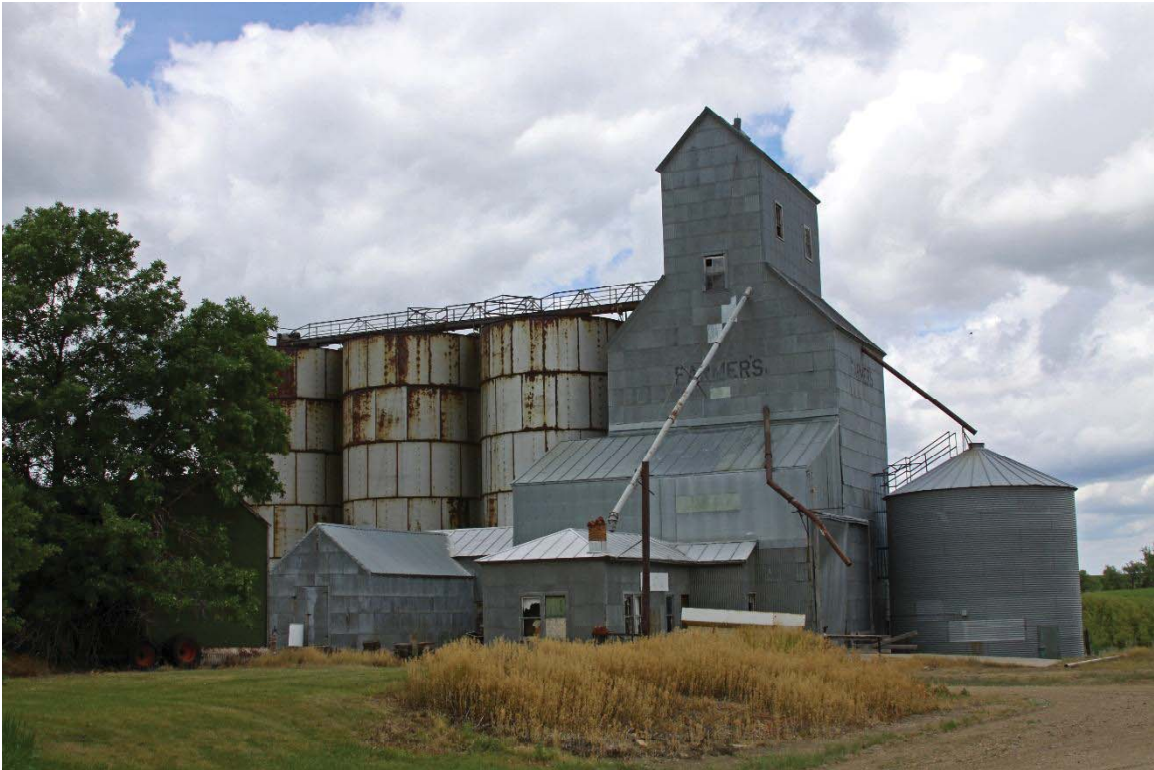
Figure 14. Site 32ML1362 grain elevator, June 18, 2019, looking north (IMG_2416.jpg).
