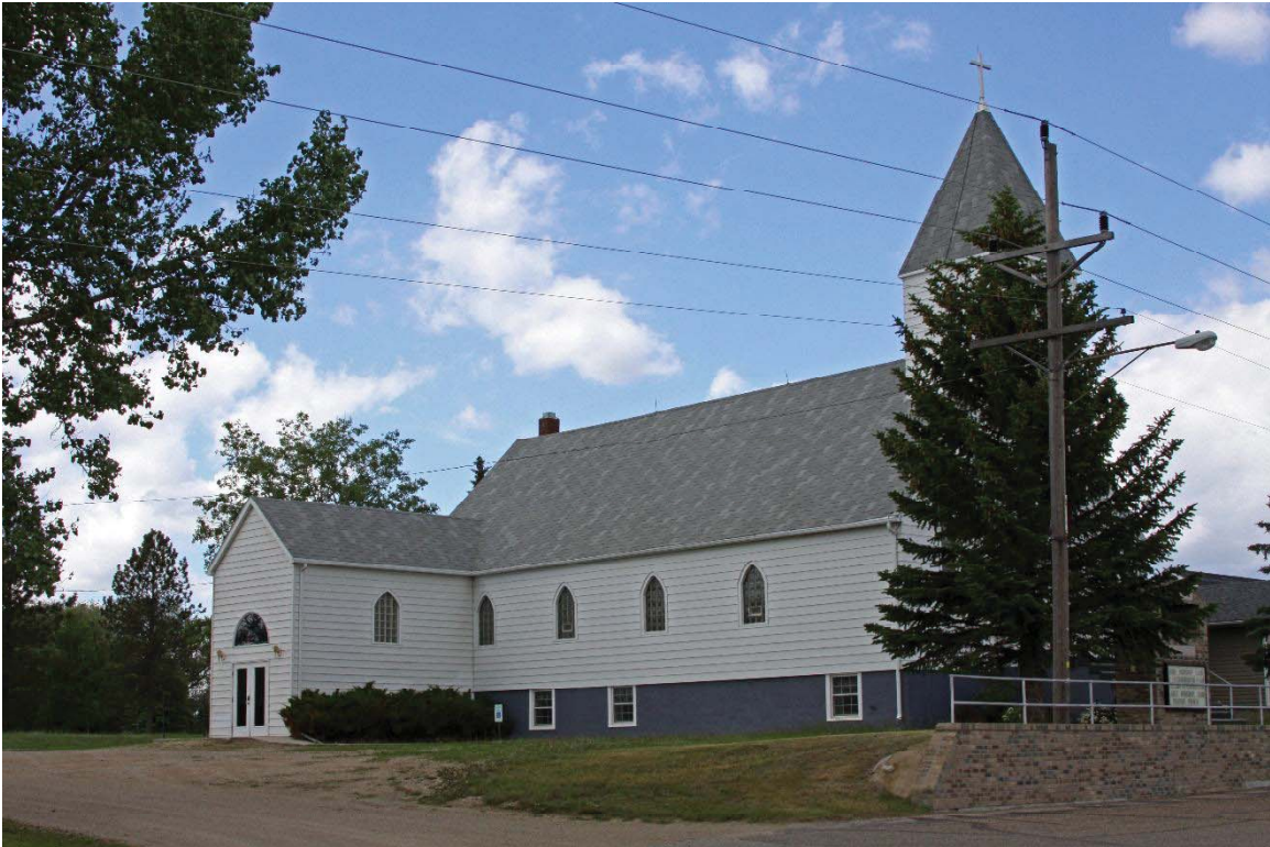
Figure 21. Site 32ML946 ineligible church, June 18, 2019, looking northwest (IMG_2584.jpg).
