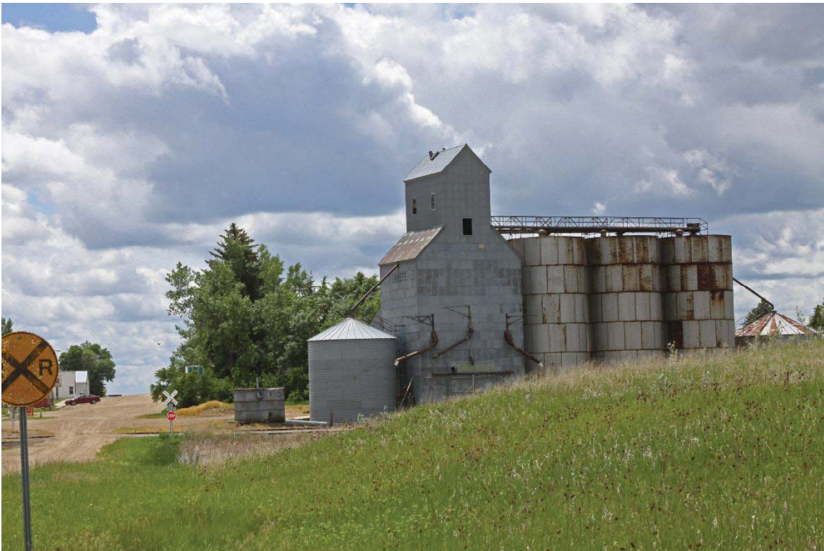
Figure 15. Site 32ML1362 grain elevator, June 18, 2019, looking south (IMG_2390.jpg).
