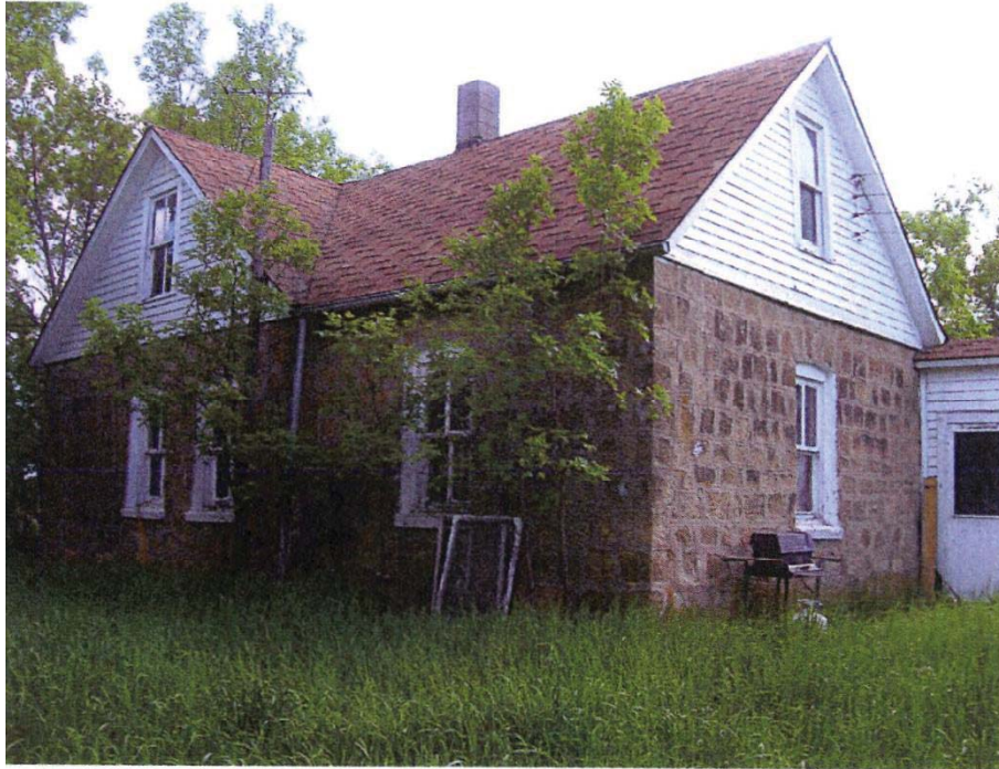
Figure 12. Site lead 32WDx747 farmhouse, photographed in 2011, looking southwest (non-BCA image; Engel 2011).
