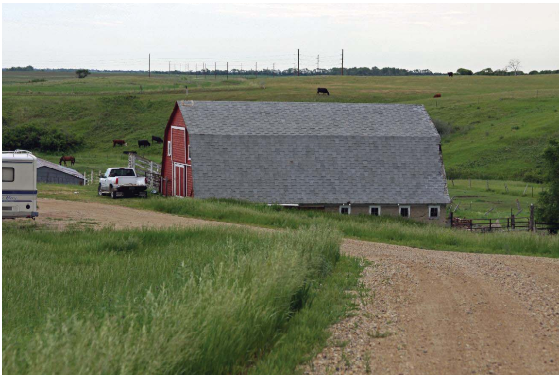
Figure 6. Site 32MH473 bank barn, June 14, 2019, facing east (IMG_1901.jpg).
