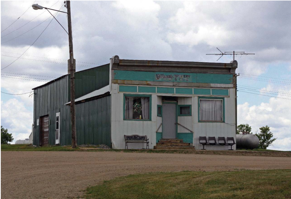
Figure 17. Site 32ML1363 Boomtown/False Front commercial building, June 18, 2019, looking west-northwest (IMG_2508.jpg).
