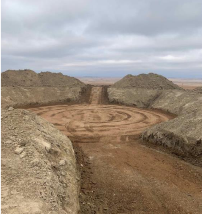
Engineered Fill Placement
