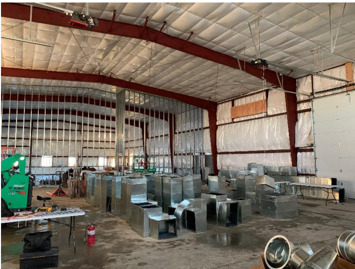
2/4/2020 O&M Building Stud Walls / HVAC Prep
