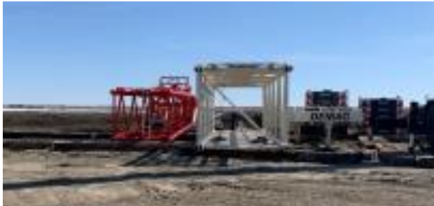
Main Crane Offload
