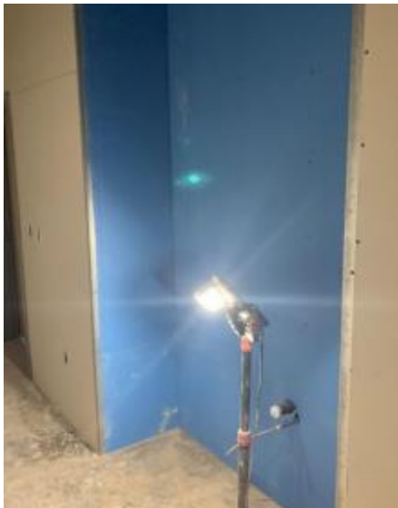
O&M Building – Drinking Fountain Rough In
