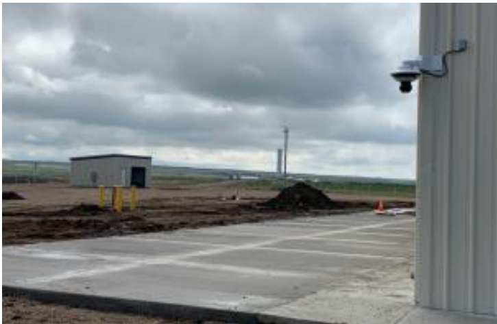
O&M Building Additional Concrete
