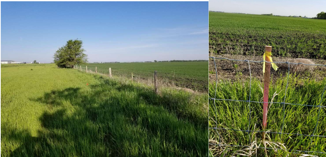
Figure 1 & 2: Above is an example of the staking on the project showing the ROW which was completed on the 14 th of May.
