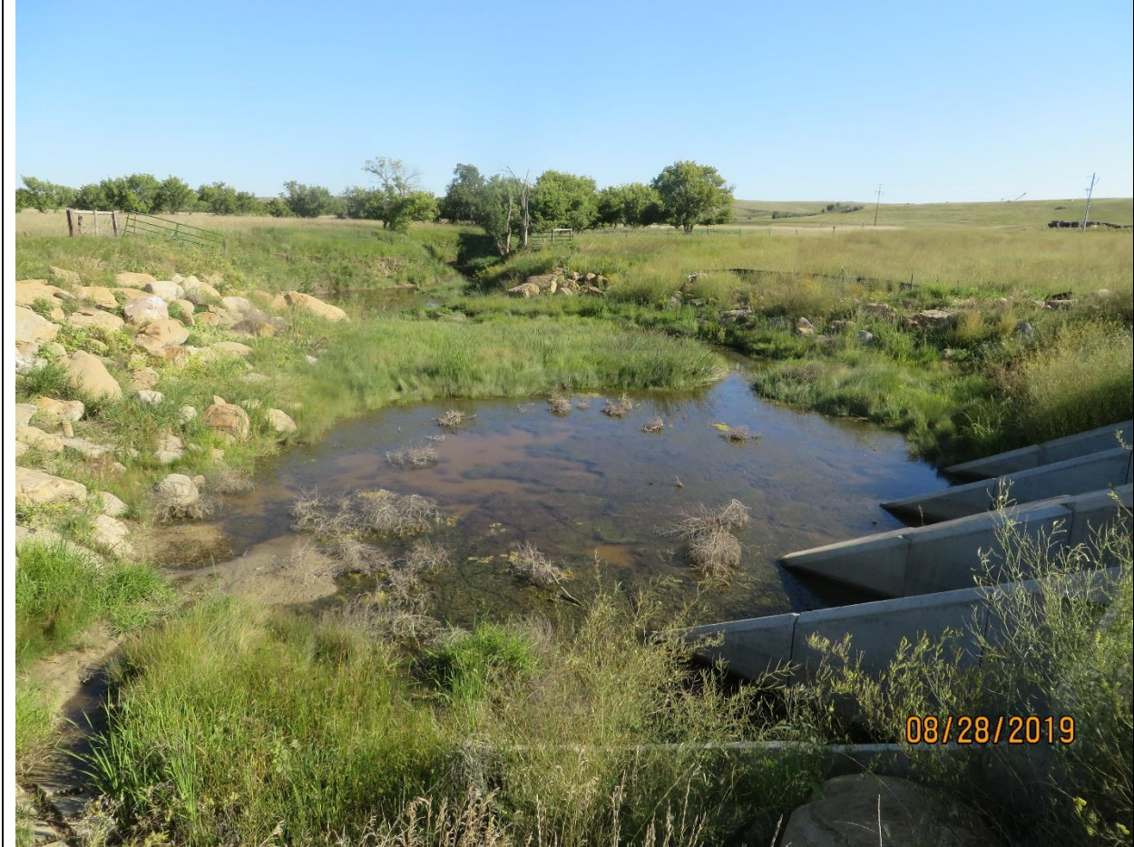
Figure 5: Small delta in stream channel north of the west of box culvert, north side of Sections 30 and 31 access road
