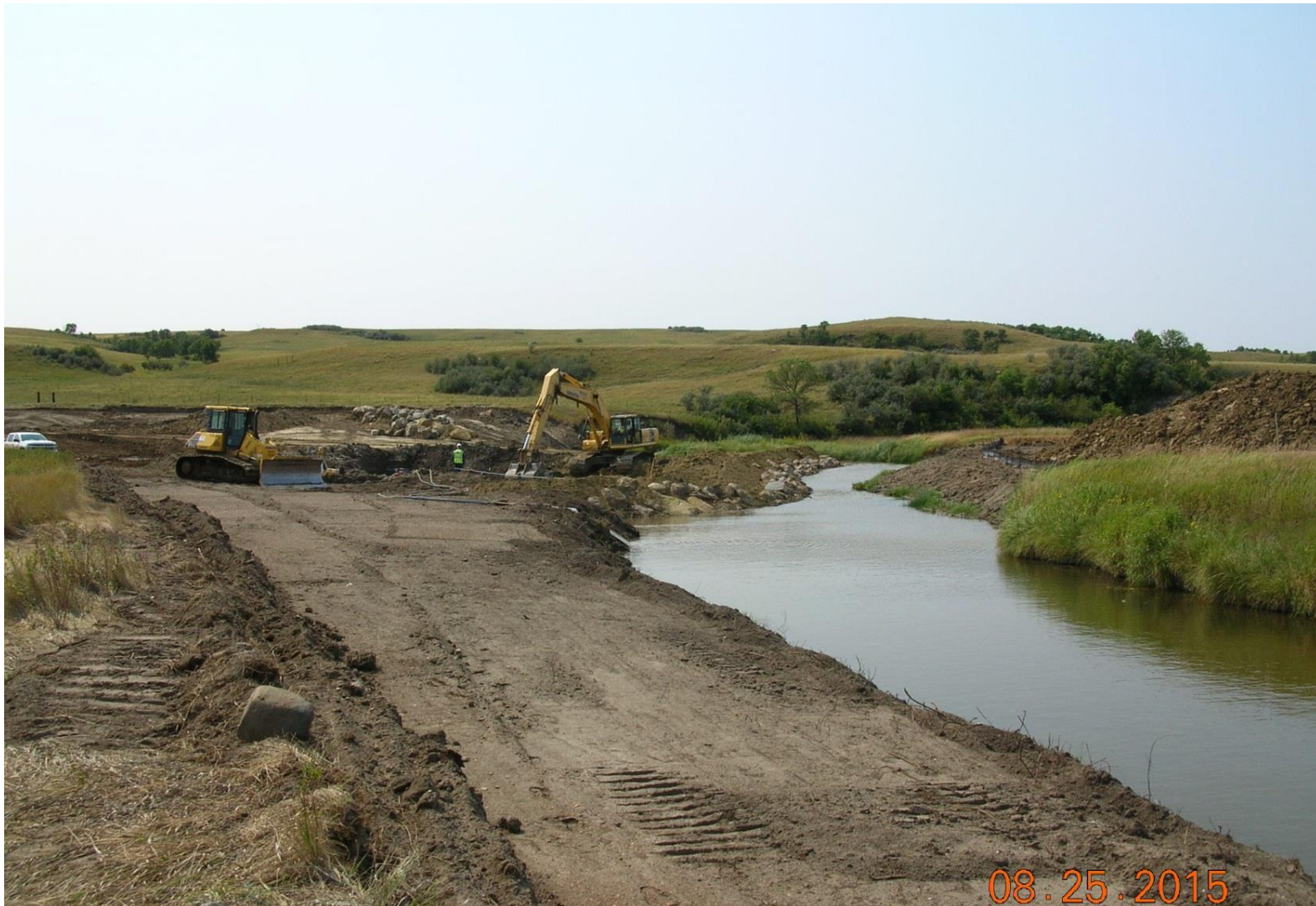
Figure 1. PC40 shovel excavating the box culvert trench along the south side of Coyote Creek for the north-south haulroad creek crossing in the SW 1 / 4 of Section 19 – facing west-southwest.
