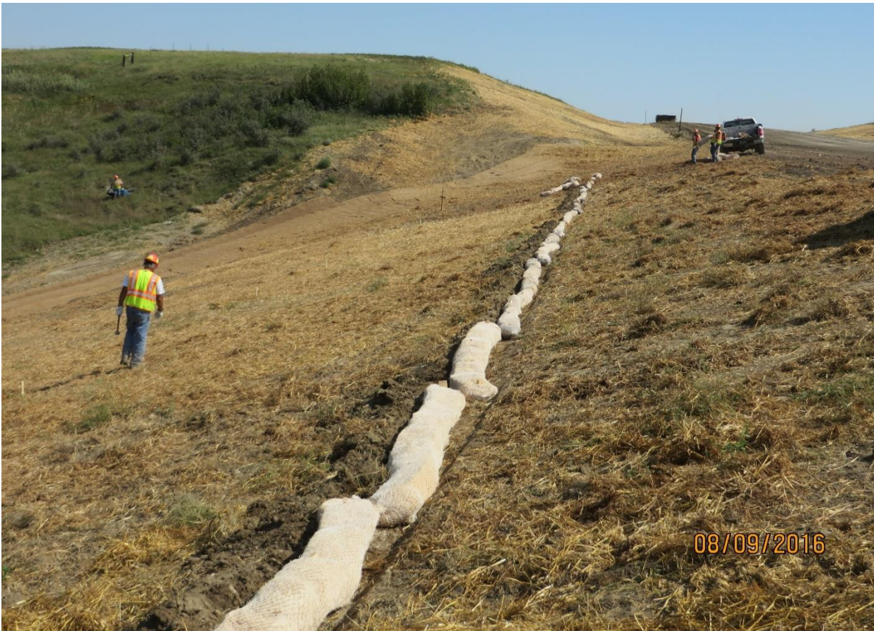
Figure 2. Installation of straw wattles at Discharge Point No. 9 in the SE1/4 of Section 8 View is toward the west
