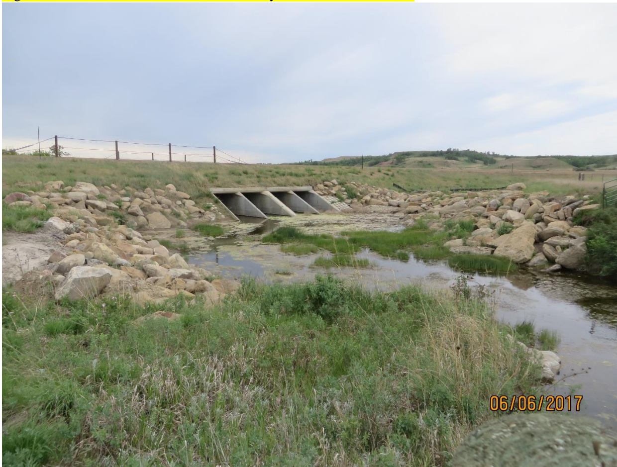
Figure 1: North end of the box culverts in Coyote Creek in Section 30
