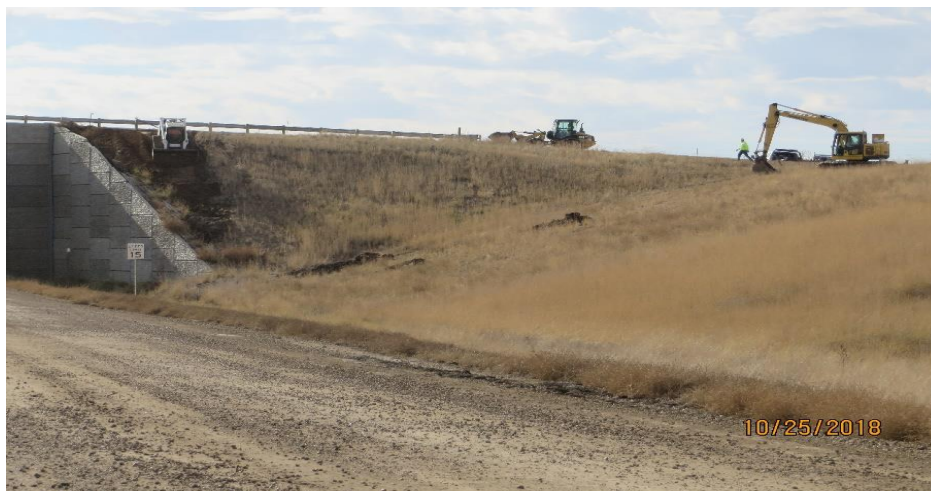
Figure 1. Erosion repair work along County Road 12 crossing
