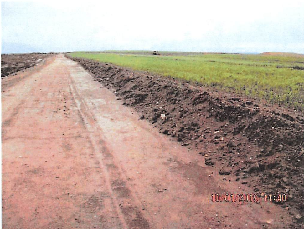
Photo 0033 Photo was taken west of the immature oat cover crop visible in Photo 0031. The flat, graded surface was SPGM subsoil. Rough-looking area in upper left corner is overburden. View north.
