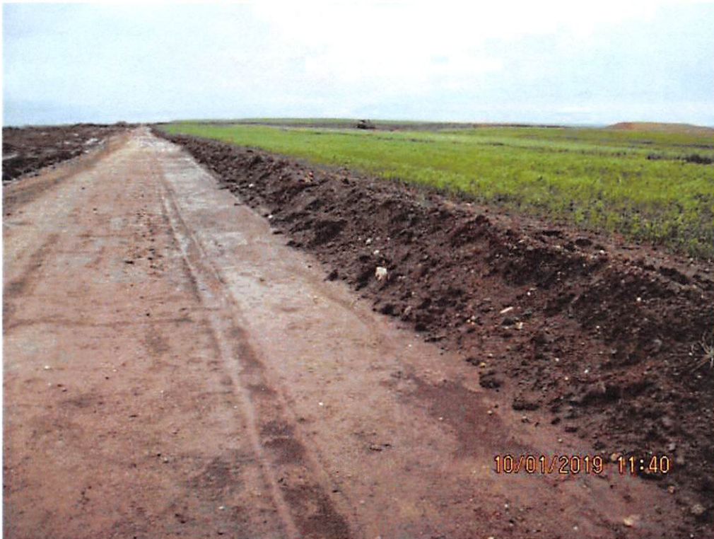
Photo 0033 Photo was taken west of the immature oat cover crop visible in Photo 0031. The flat, graded surface was SPGM subsoil. Rough-looking area in upper left corner is overburden. View north.
