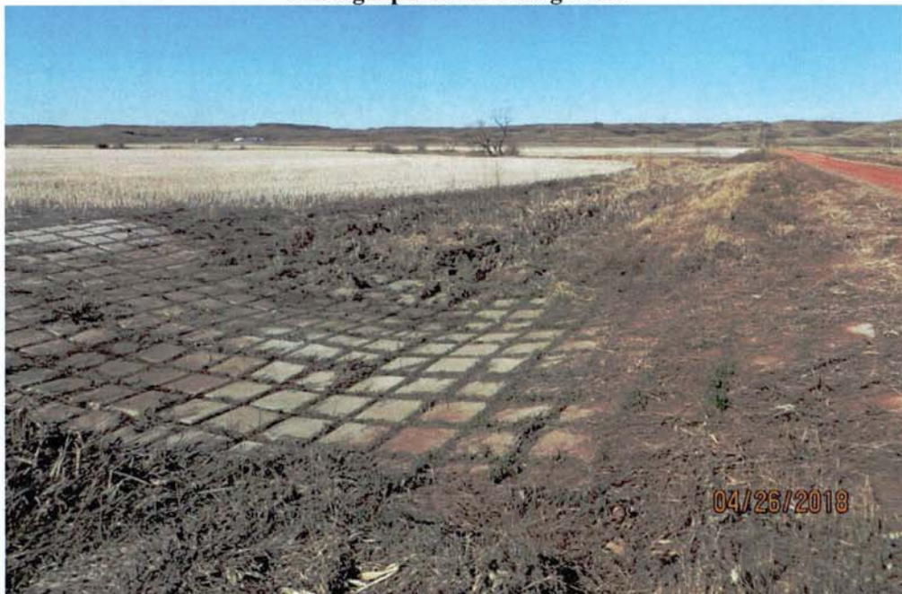
Figure 3. Flexcrete crossing in the road ditch on the north side of the NW¼ of Section 34. Photograph taken facing west.
