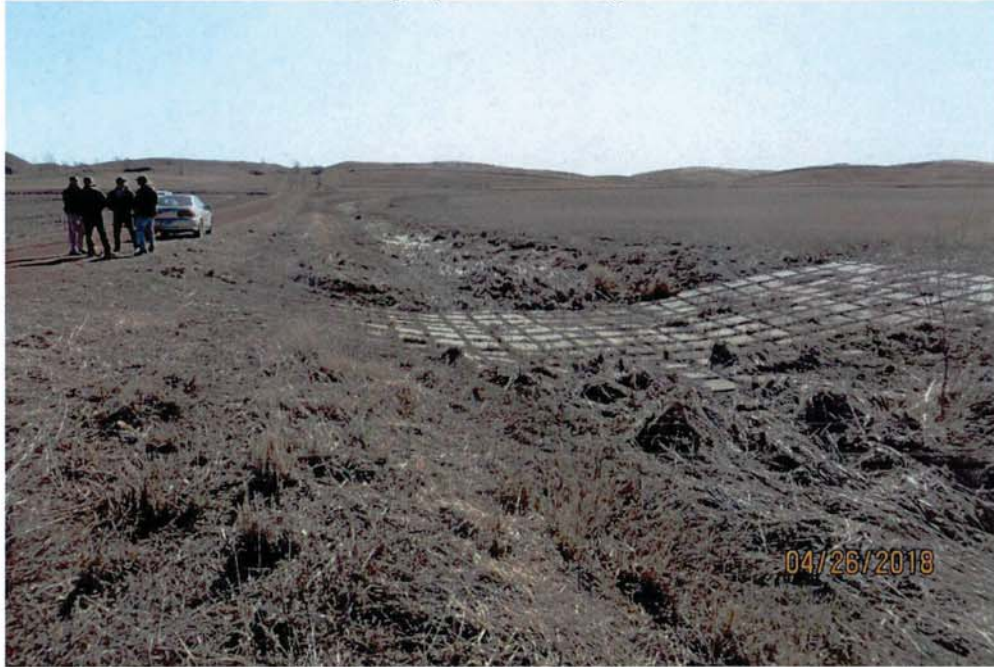
Figure 2. Flexcrete crossing in the road ditch on the north side of the NW¼ of Section 34. Photograph taken facing east.
