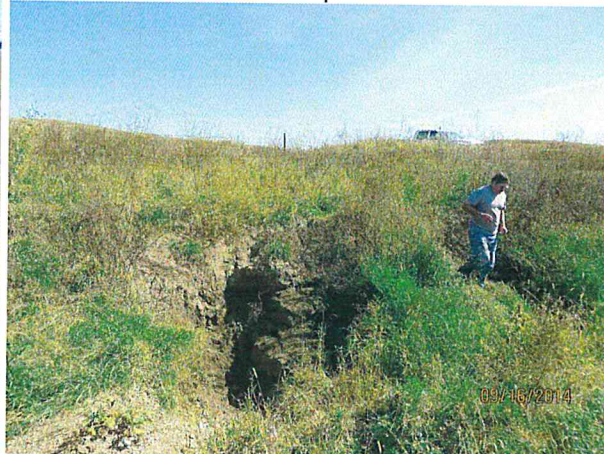
Diversion ditch on 16 Sep 2014
