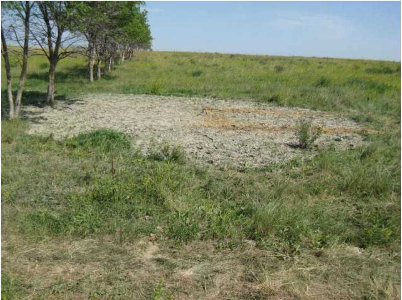
Figure 2. Typical Surface Expression of a Frac-Out
